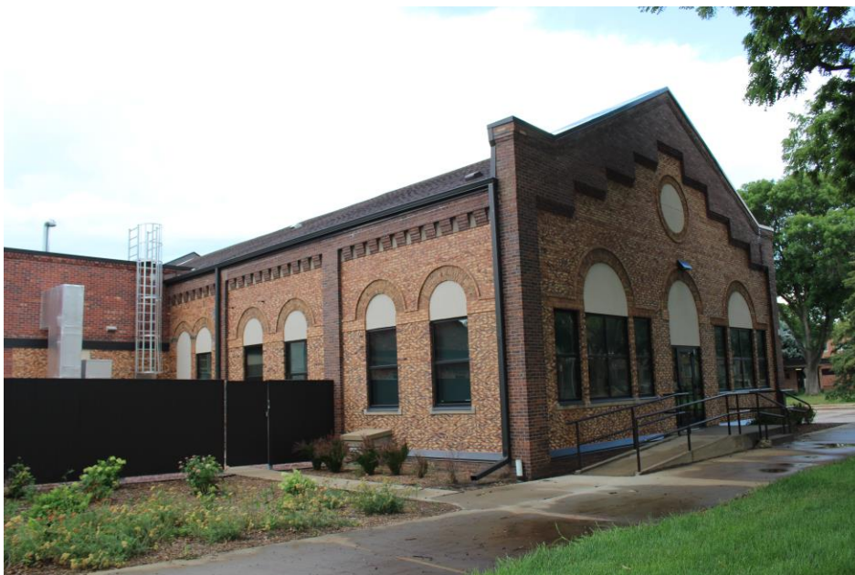
5. Old Power Plant, south and west wings, southwest corner (camera facing northeast)
