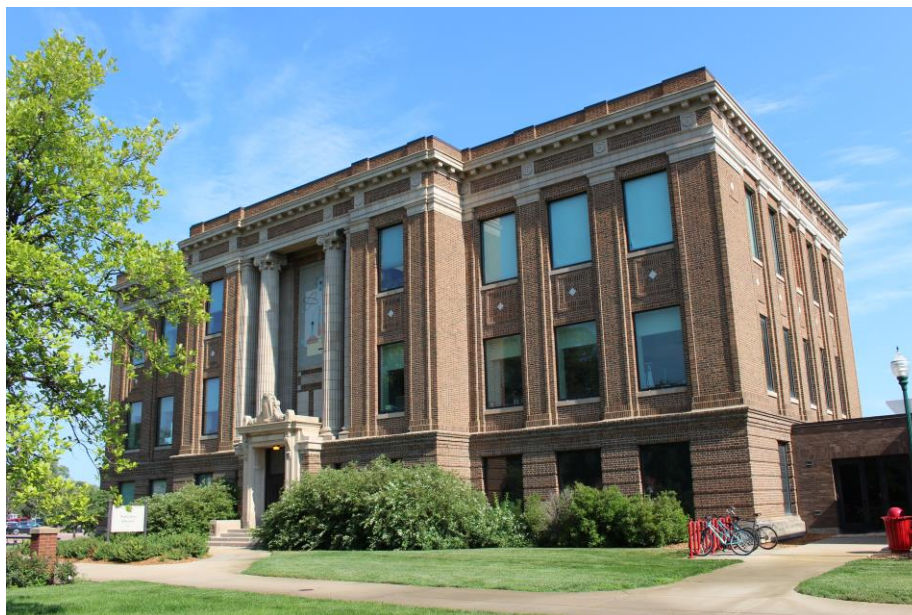
7. Chemistry Building, front (south) elevation (camera facing northwest)
