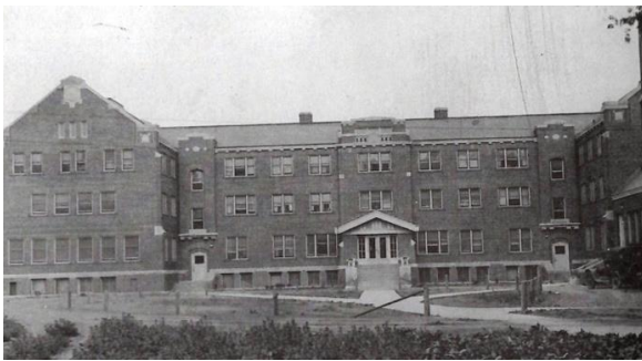
Dakota Hall, (built 1918-19) (photo from Tour of The University of South Dakota's Historic Buildings)
