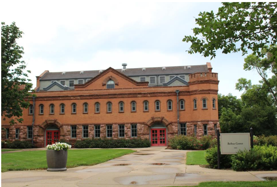
3. Armory/Gymnasium (Old), south elevation (camera looking north)
