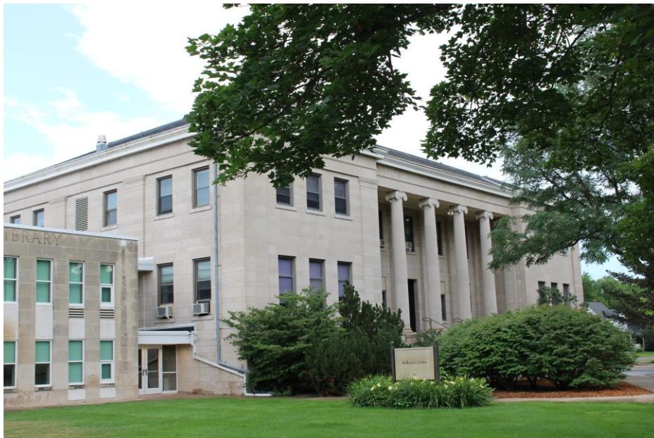
4. College of Law, front elevation from northwest corner (camera facing southeast)
