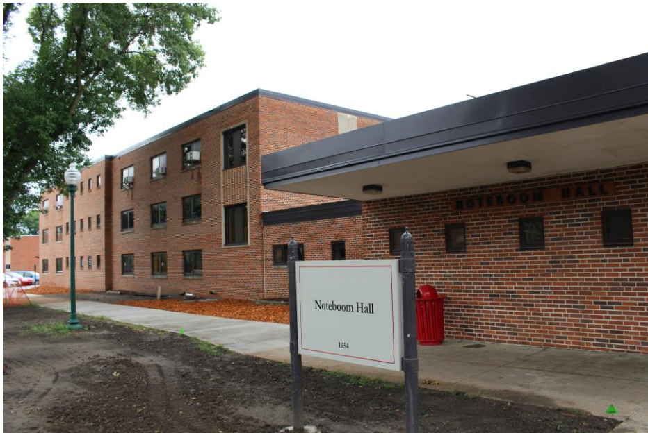
12. Charlotte Noteboom Hall, front (south) elevation (camera facing northwest)
