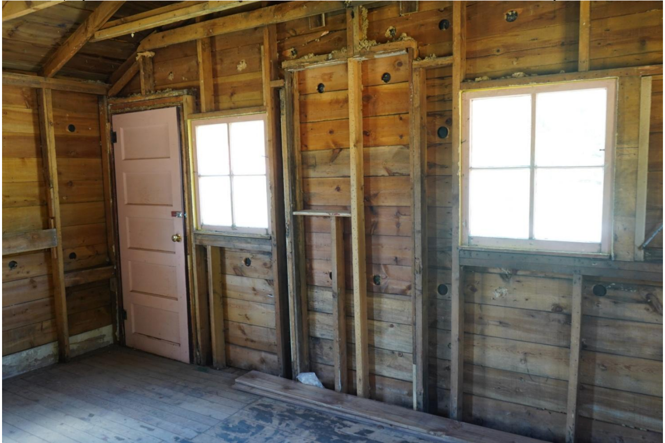
SD_PenningtonCounty_CampF-4Pactola ConservationCorpsBarrack_0007. Interior view.
