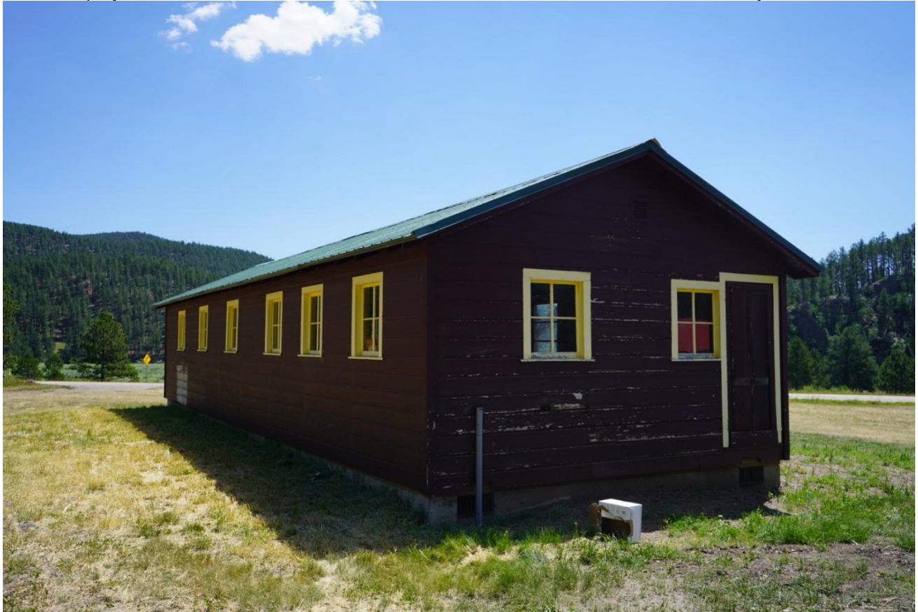
SD_PenningtonCounty_CampF-4Pactola ConservationCorpsBarrack_0003. Looking southeast at west and north elevation.
