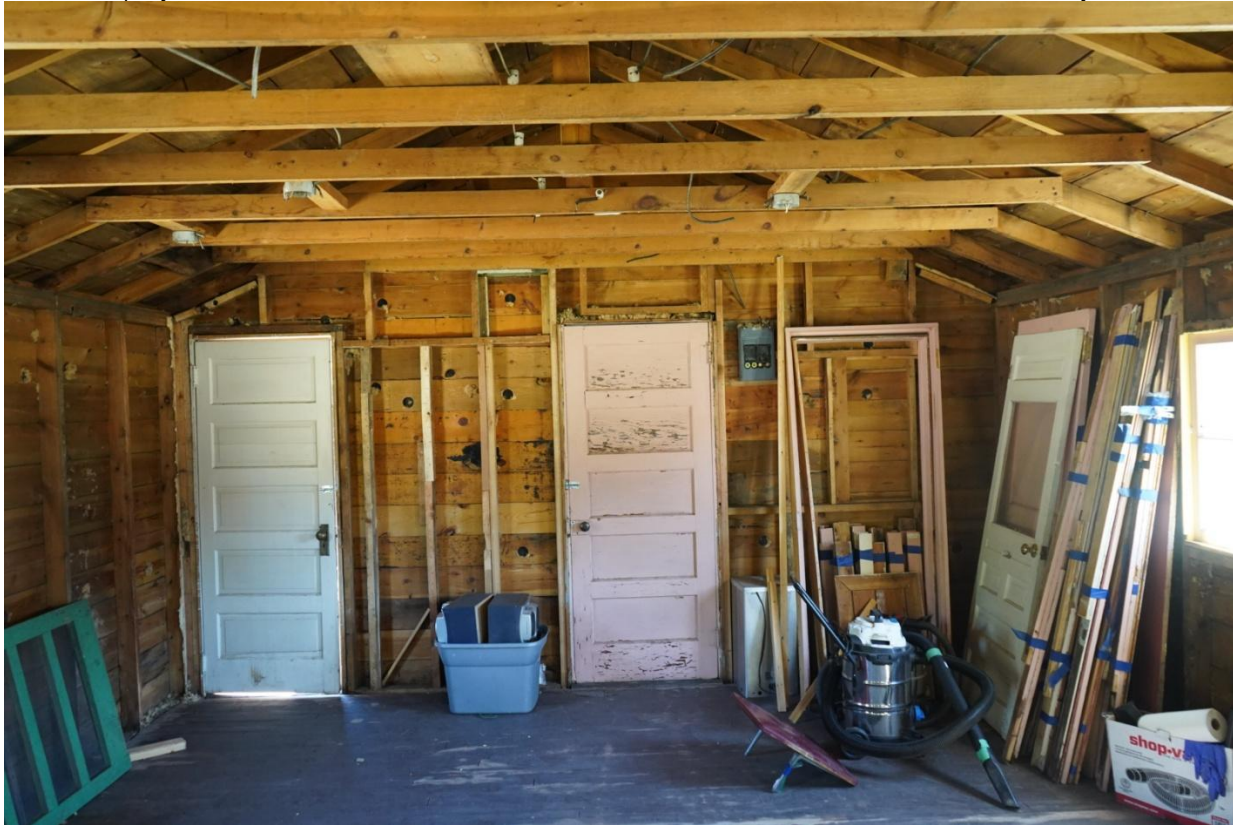
SD_PenningtonCounty_CampF-4Pactola ConservationCorpsBarrack_0008. Interior view.
