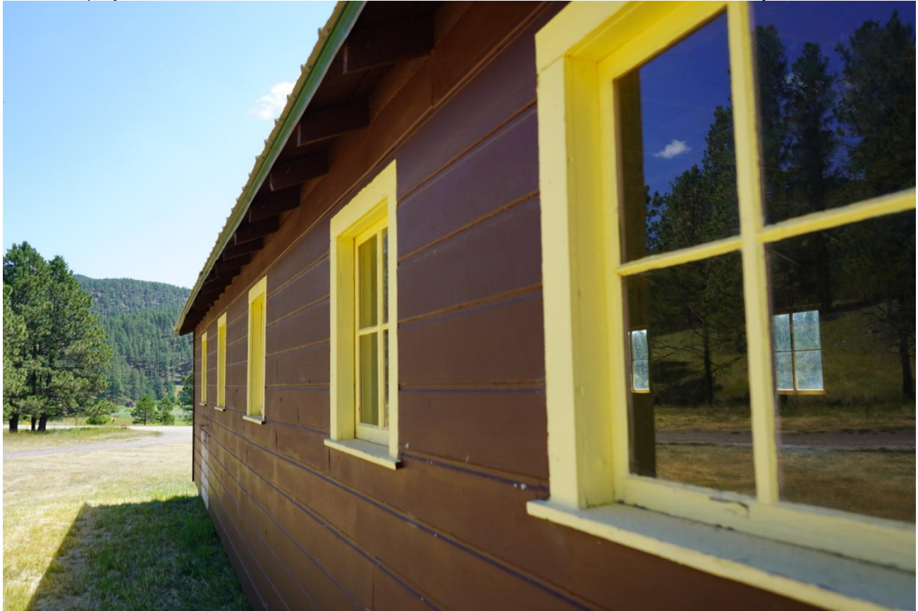
SD_PenningtonCounty_CampF-4Pactola ConservationCorpsBarrack_0005. Looking southeast at north elevation.
