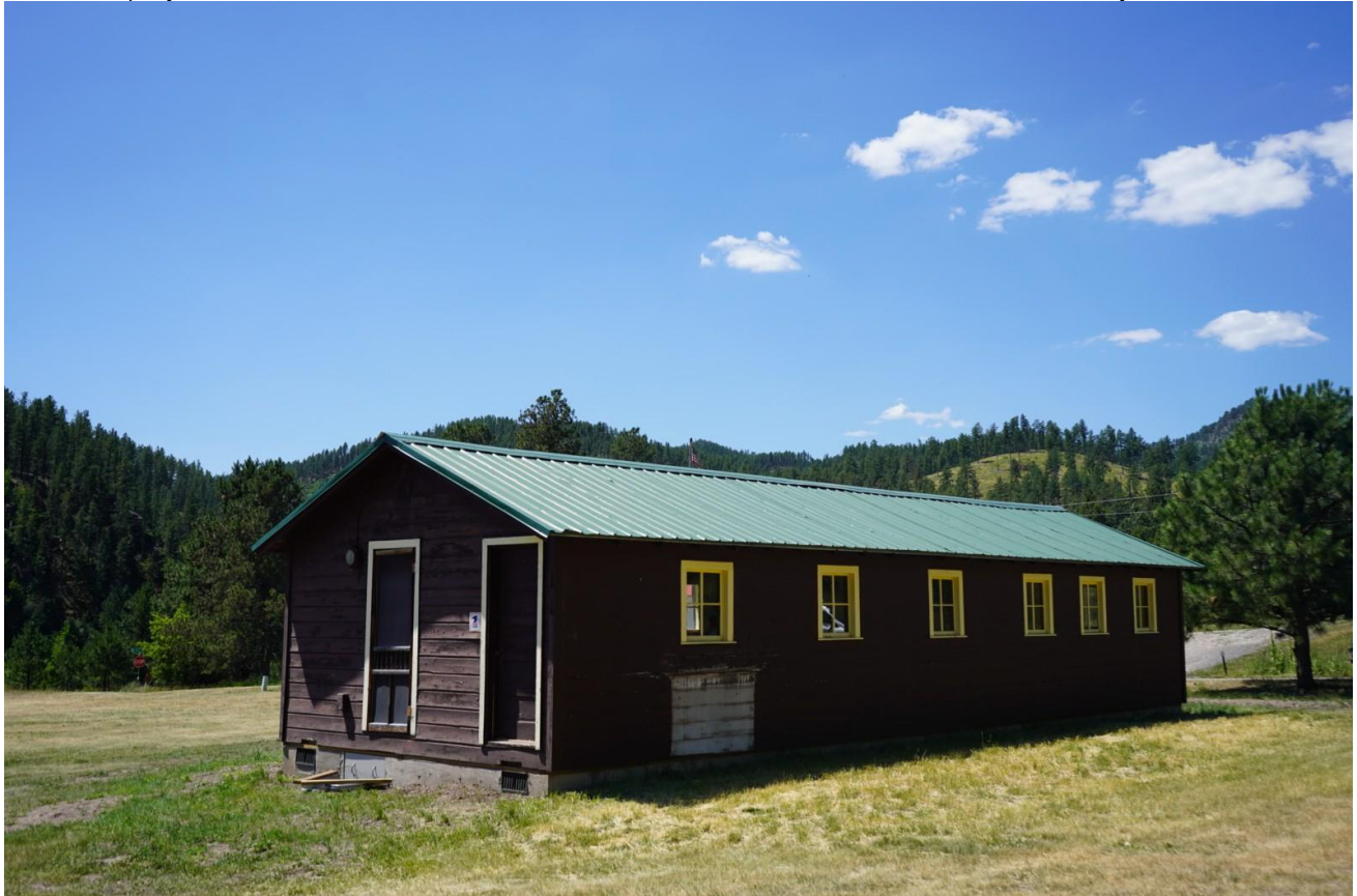
SD_PenningtonCounty_CampF-4Pactola ConservationCorpsBarrack_0002. Looking southwest at north and east elevation.
