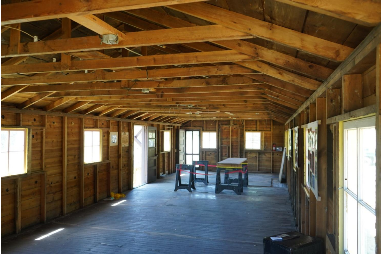
SD_PenningtonCounty_CampF-4Pactola ConservationCorpsBarrack_0006. Interior view.
