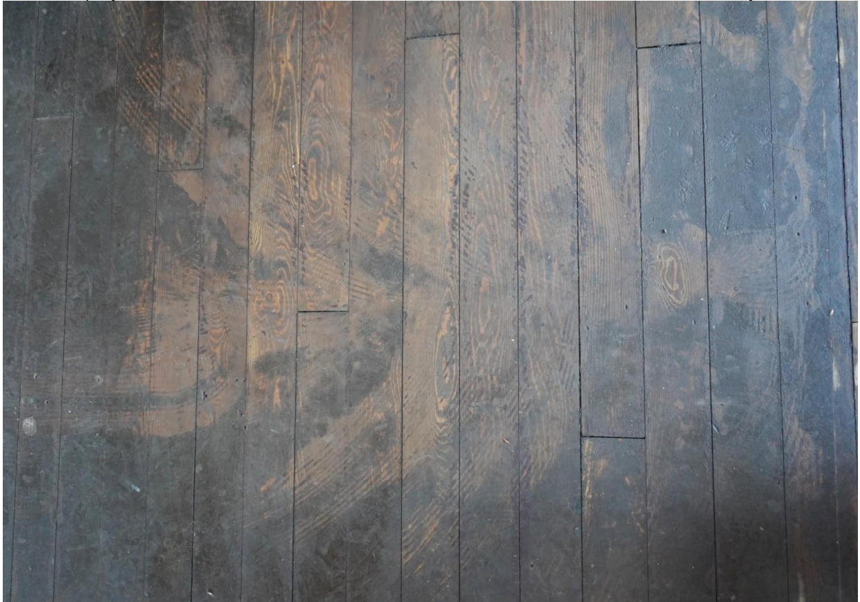
SD_PenningtonCounty_CampF-4Pactola ConservationCorpsBarrack_0009. Interior floor.
