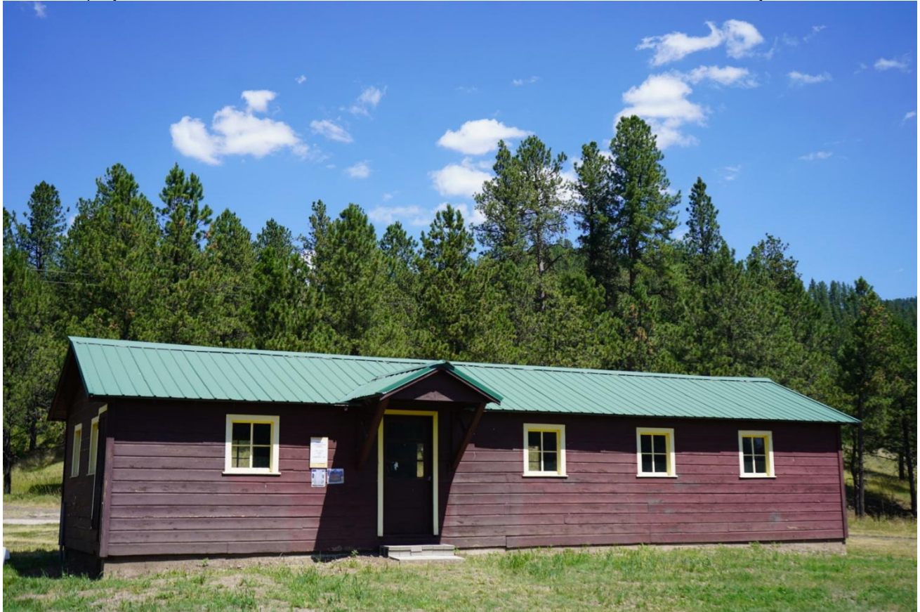
SD_PenningtonCounty_CampF-4Pactola ConservationCorpsBarrack_0001. Looking north at south elevation.
