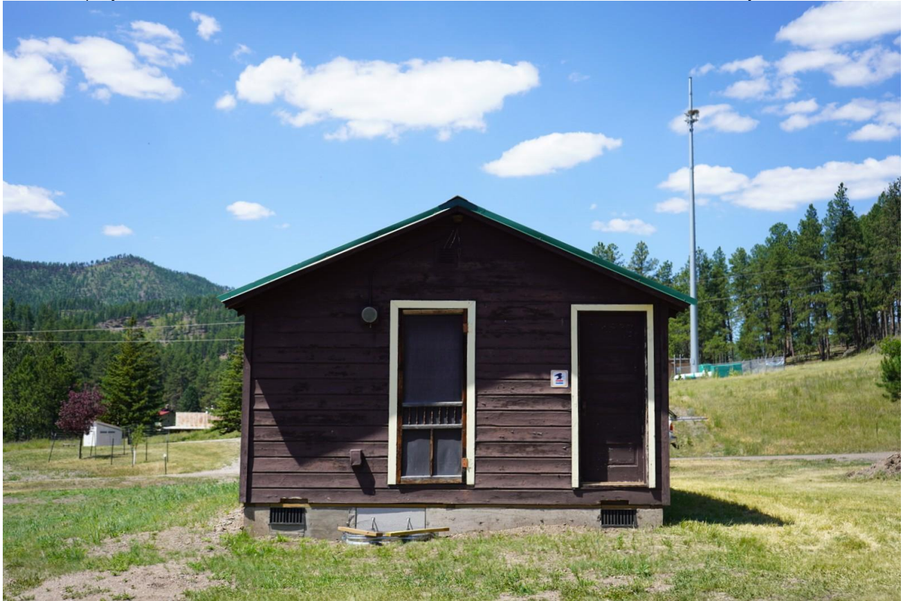
SD_PenningtonCounty_CampF-4Pactola ConservationCorpsBarrack_0004. Looking west at east elevation.
