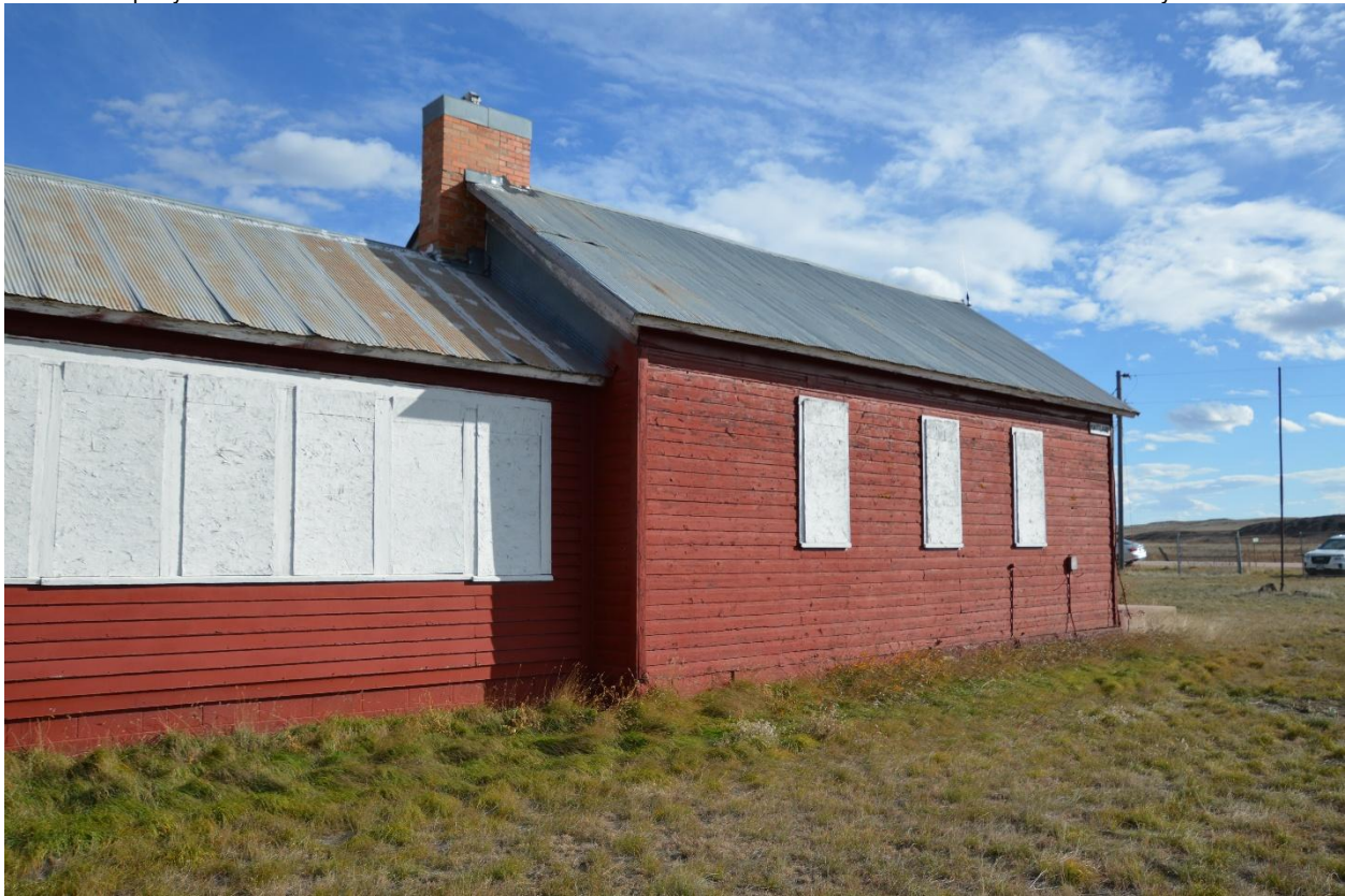
SD_MaitlandSchoolhouse_FallRiverCounty_0003. Looking SE at W elevation.
