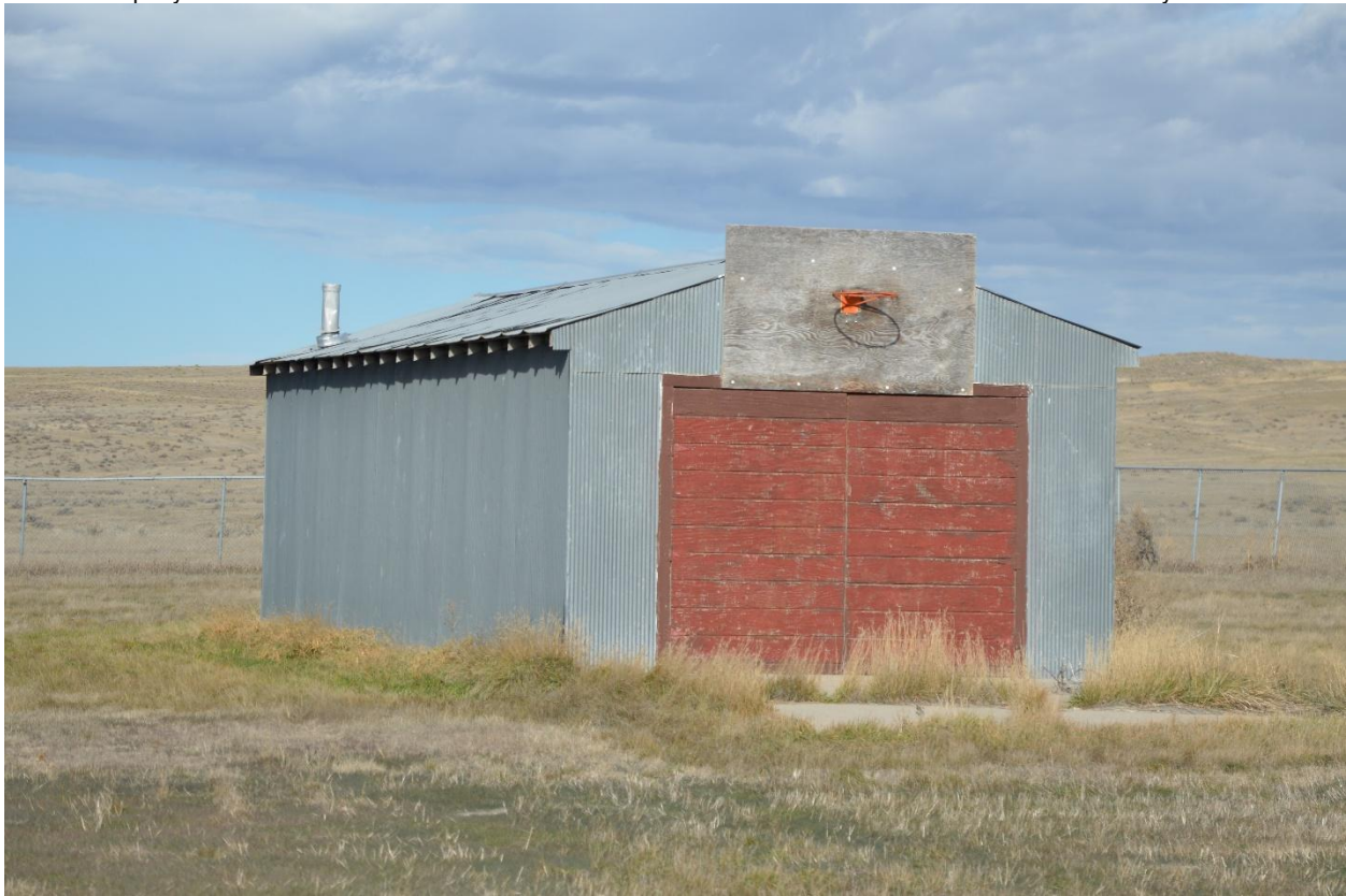
SD_MaitlandSchoolhouse_FallRiverCounty_0009. Looking NE at S and W elevations of horse barn/garage.
