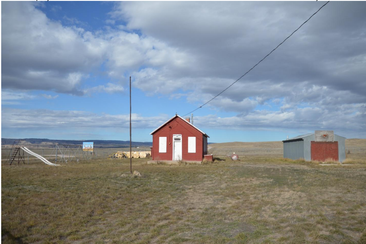
SD_MaitlandSchoolhouse_FallRiverCounty_0005. Looking N at S elevation and playground.
