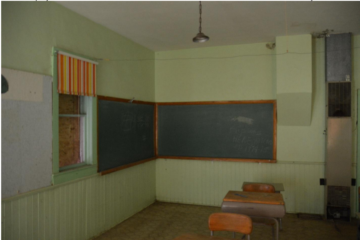
SD_MaitlandSchoolhouse_FallRiverCounty_0007. Interior of 1892 volume.
