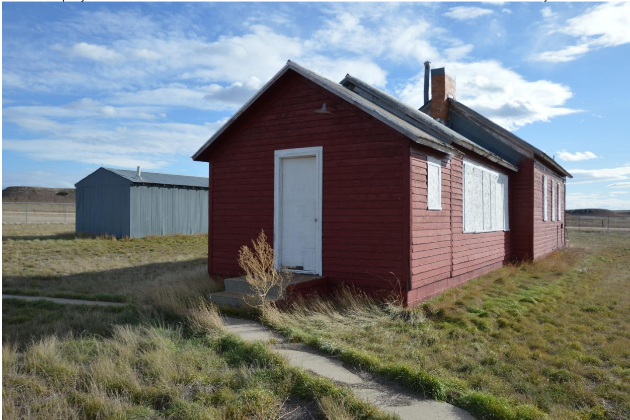
SD_MaitlandSchoolhouse_FallRiverCounty_0004. Looking SE at N and W elevations.
