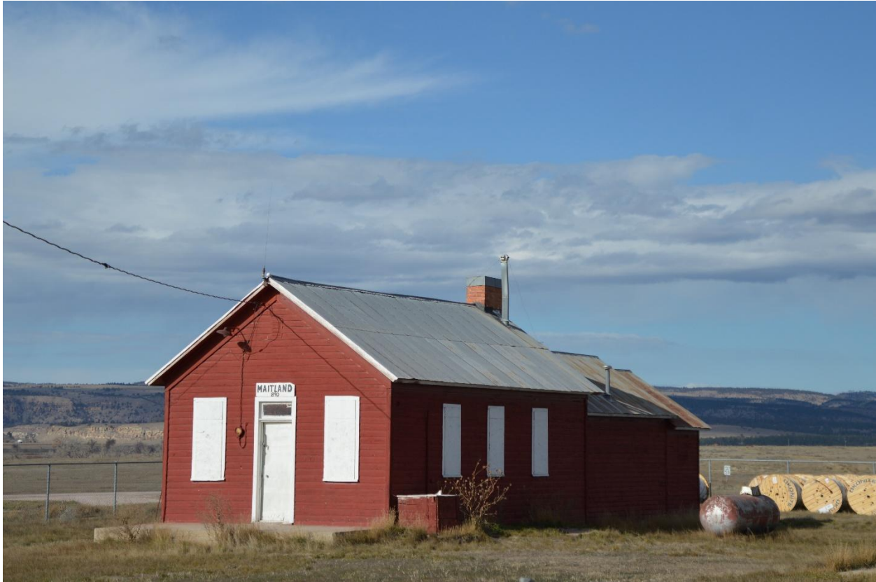
SD_MaitlandSchoolhouse_FallRiverCounty_0001. Looking NW at S and E elevations.
