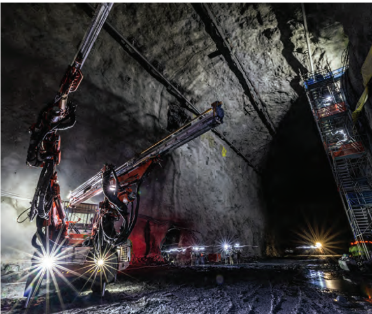
Top: A mucker on the left and jumbo drill on the right as seen from directly above in the north DUNE Cavern.
