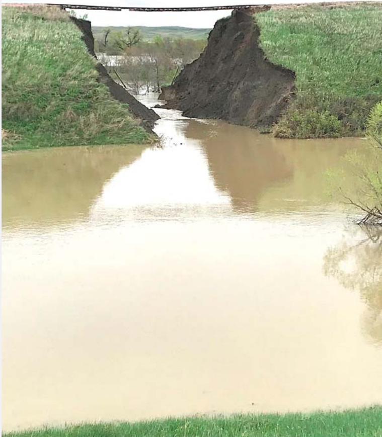
Capa, South Dakota on May 22, 2019 Washout (left) and Repair (right)
