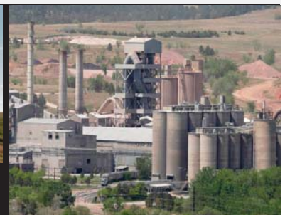
GCC – Kiln Expansion
