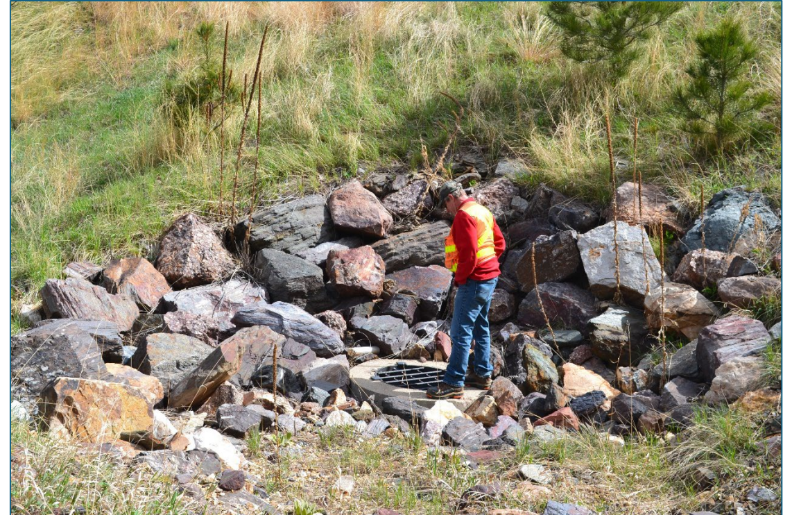
Stormwater control facility inspection, May 2026
