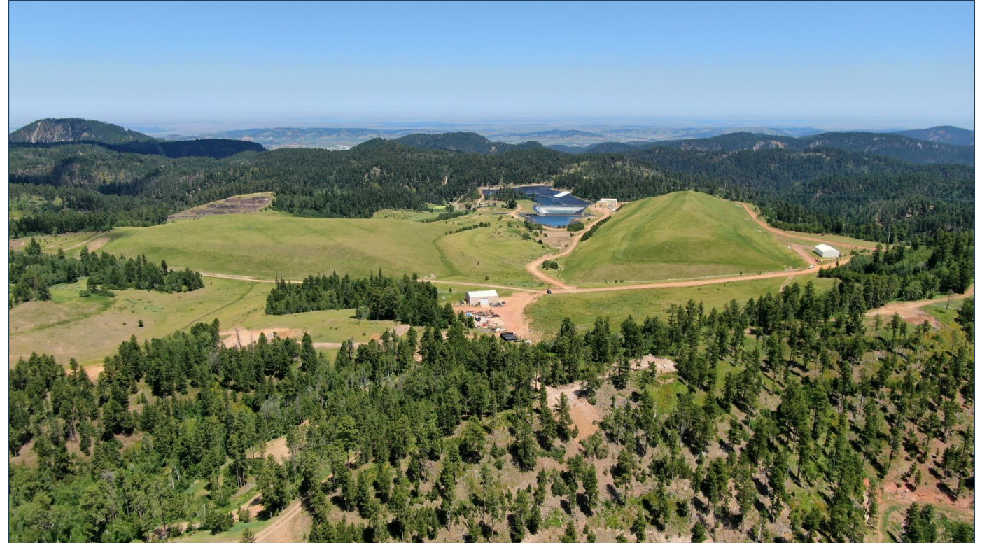
Capped and reclaimed leach pads, Richmond Hill Mine
