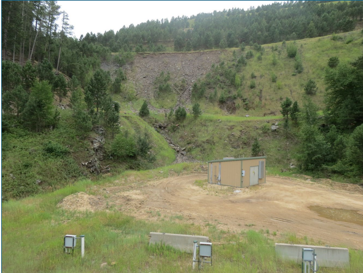
East Ravine area prior to 2024 repairs
