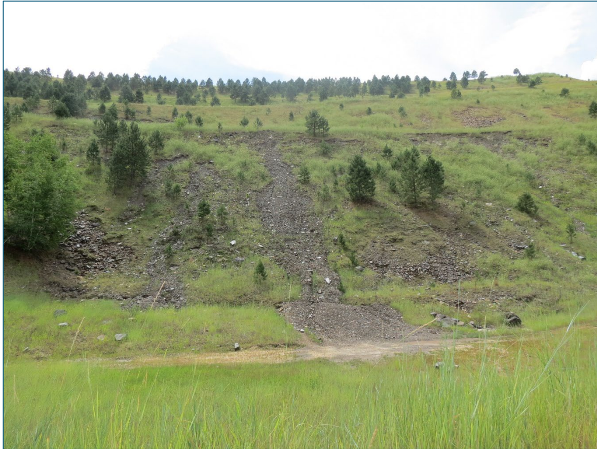
Soil slump in Blacktail area prior to 2024 repairs
