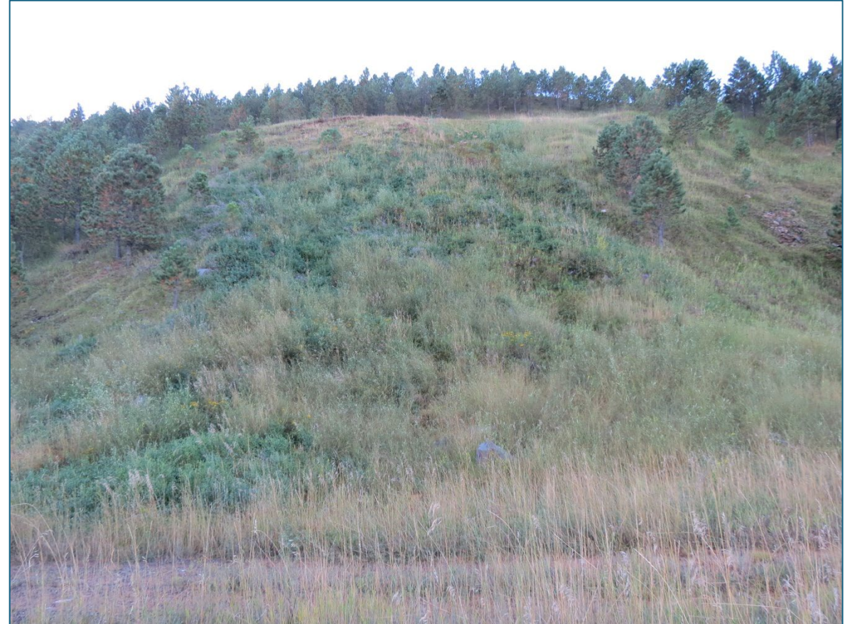
Repaired area showing reestablished vegetation (fall 2025 photo)
