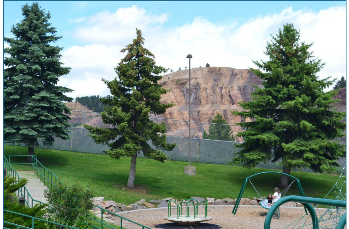
Safety fence near Open Cut, Manuel Brothers Park, Lead
