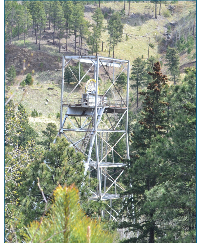
No. 5 Shaft Headframe, SD Science and Technology Authority, 2026
