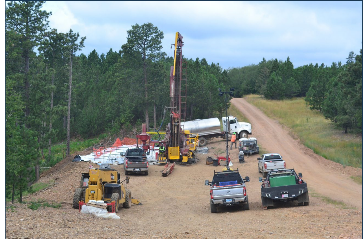
Dakota Gold groundwater monitoring well installation, 2025
