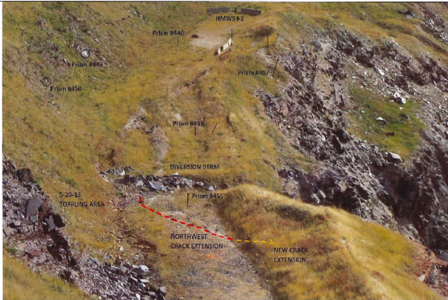
ACCESS ROAD MOVEMENTS: SE VIEW OF EAST BLOCK (PHOTOGRAPH TAKEN ON OCTOBER 23, 2018)
