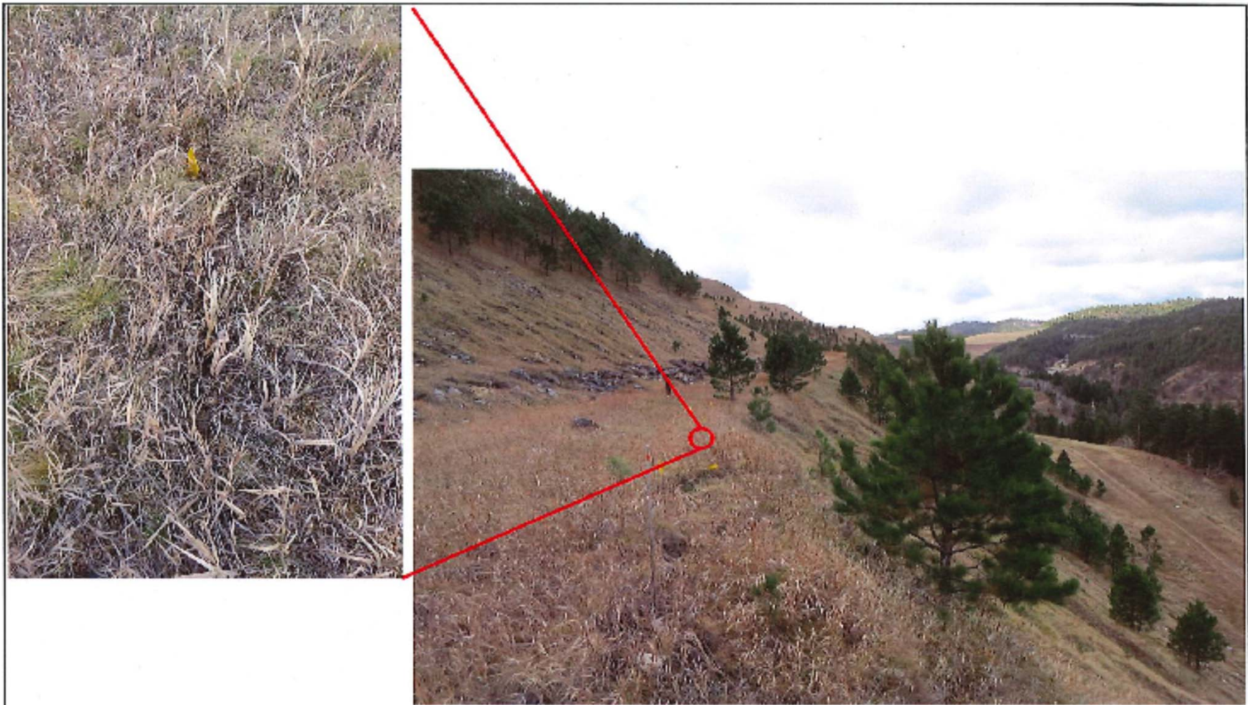
TENSION CRACK AT THE CREST OF THE 5100 BENCH IN GAYVILLE GULCH LOOKING WEST (PHOTOGRAPH TAKEN ON OCTOBER 30, 2018)
