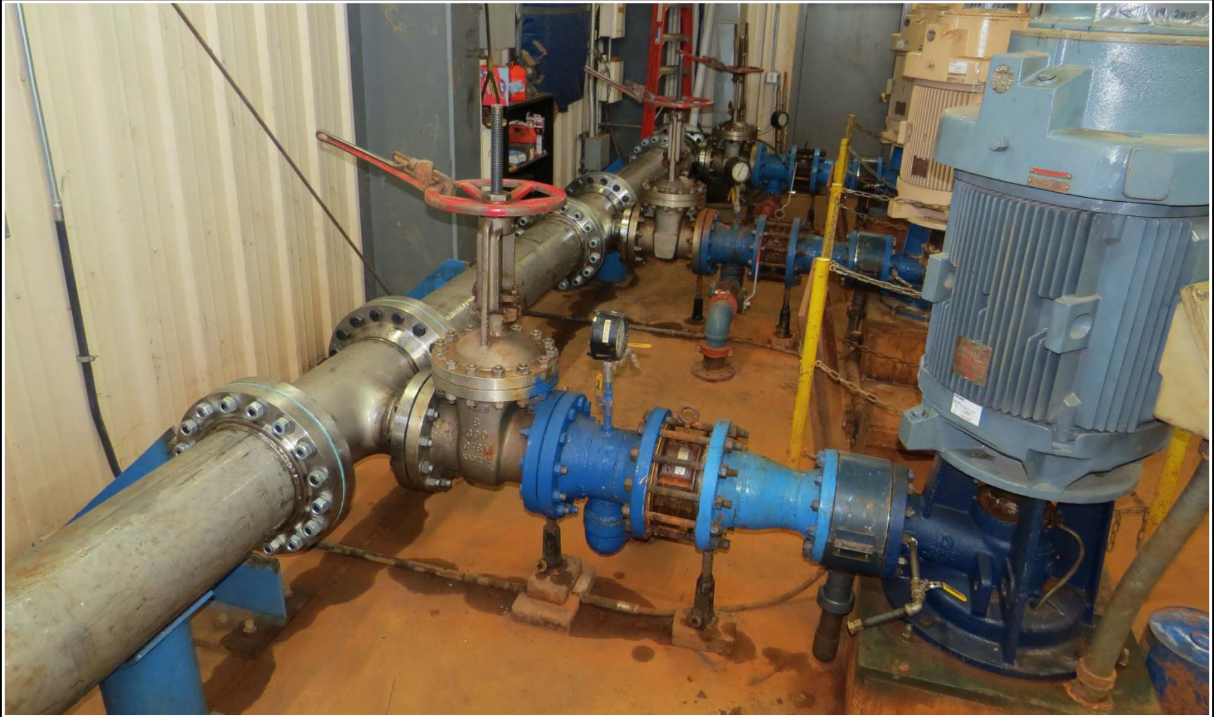
Stainless Steel Header at Seepage Collection
