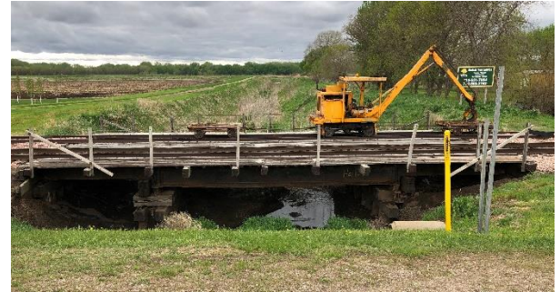
Figure 2: T512.5 main line and auxiliary track facing west.
