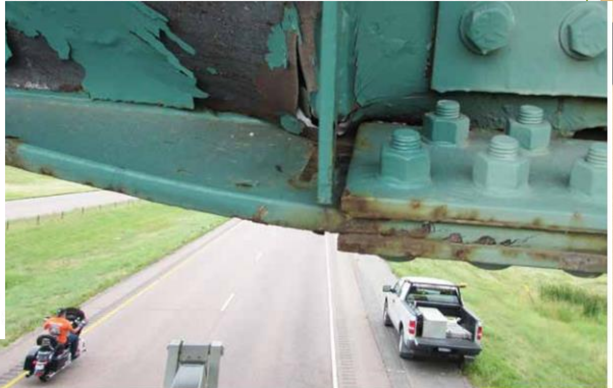
Above: A steel girder on the Hartford exit overpass damaged by an Aug. 2016 hit. Right: Damage to the same bridge in 2016. The total for heat straightening steel girders, and replacing other bridge parts for both
