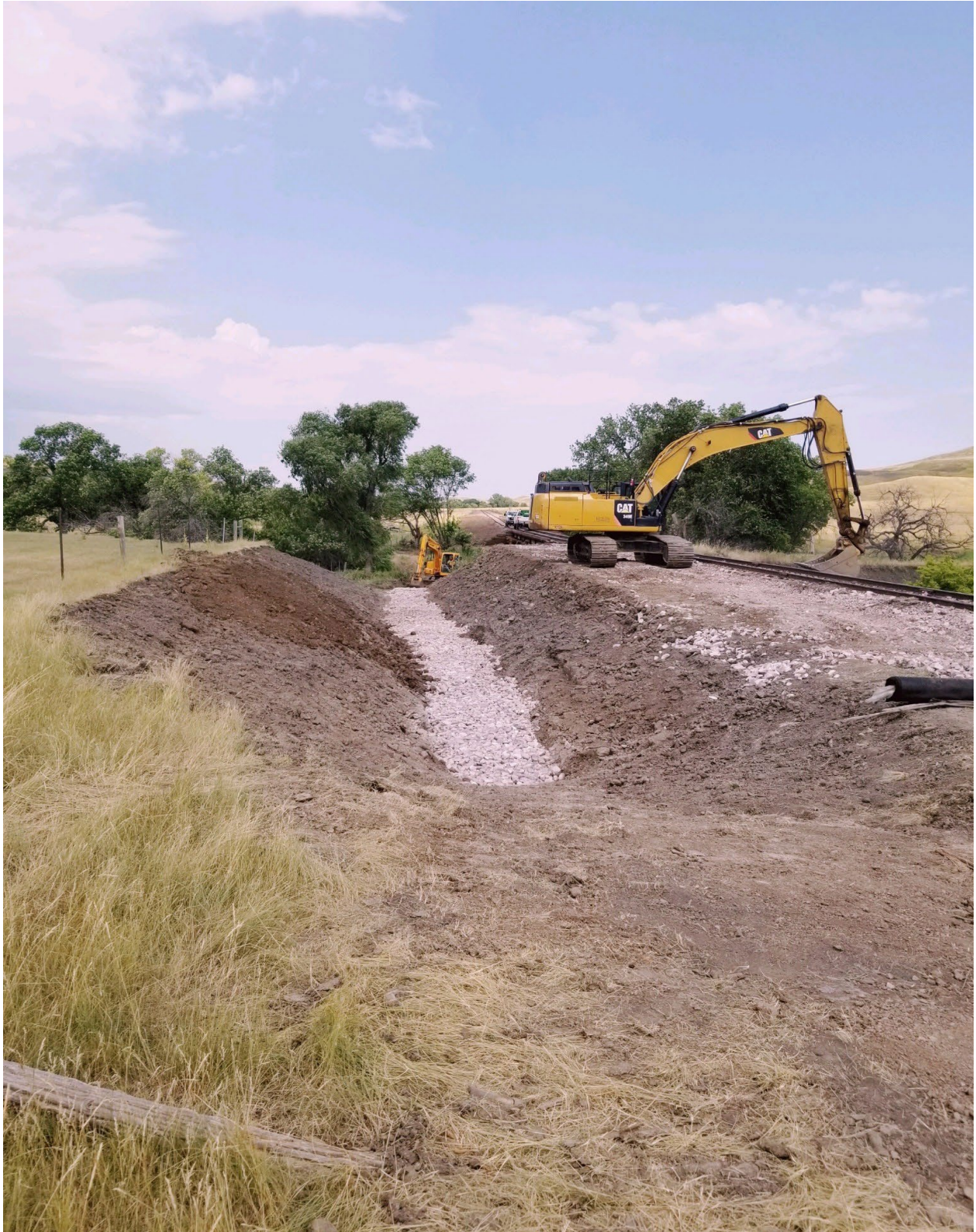
Mp 448.5 French drain installation 8-25-22
