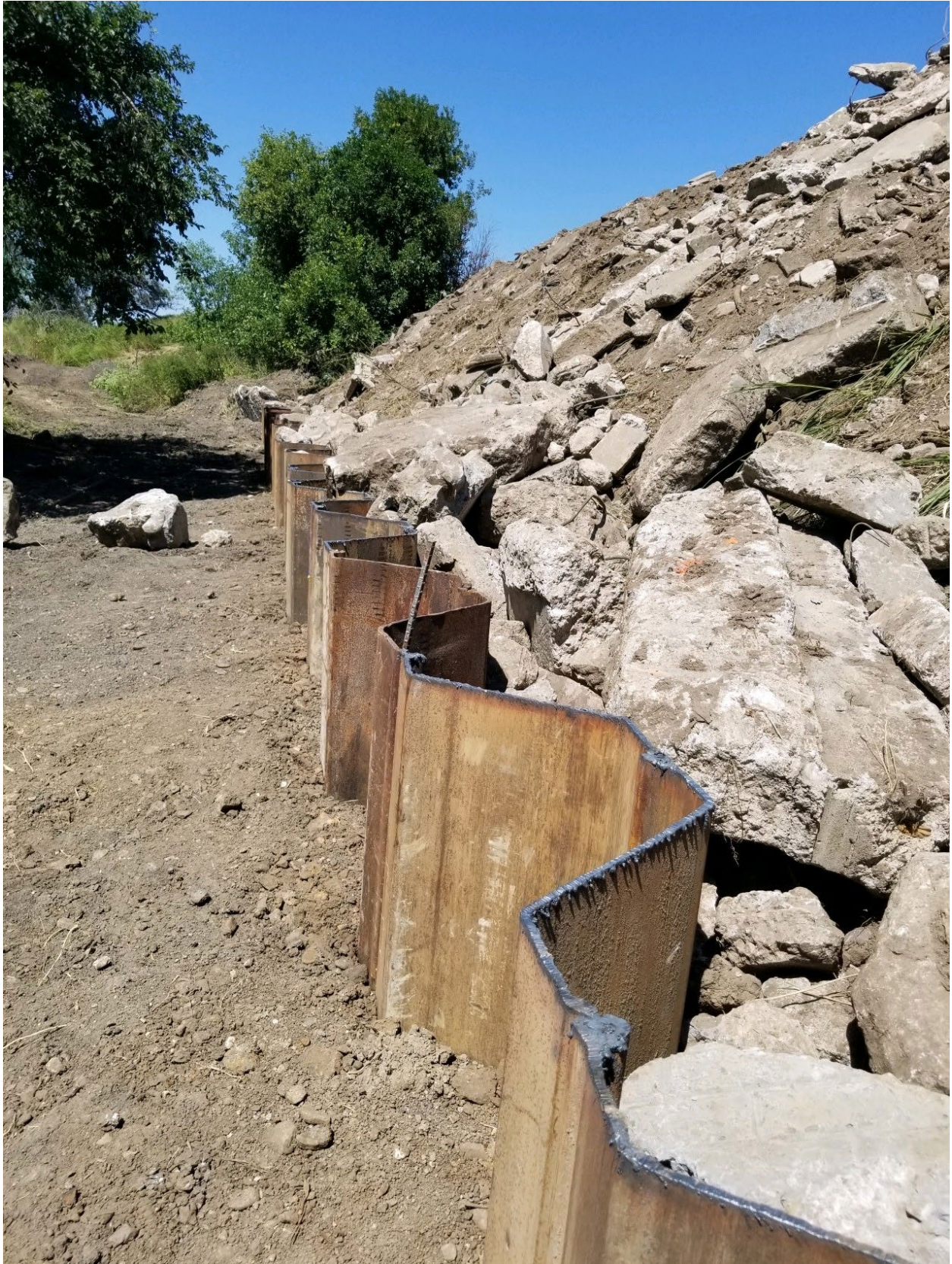
Sheet pile and embankment repair 8-10-22
