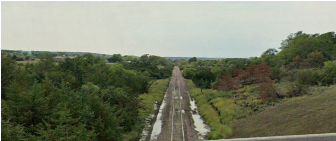
Drainage issues along American Creek – project area to be undercut
