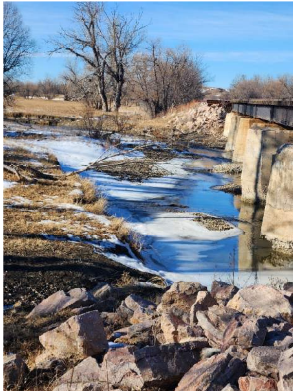
CDI_Channel Looking Southwest Upstream of Bridge at MP 617.30
