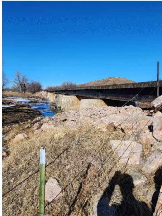
CDI_Profile Structure 617.30 Looking Northwest
