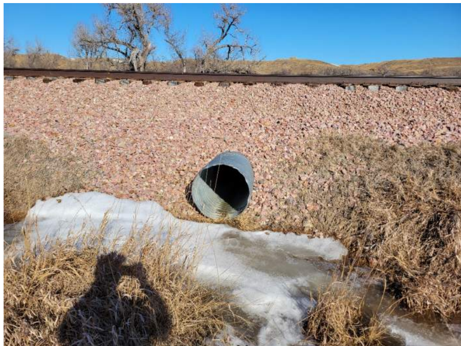
CDI_Upstream End of Existing 24" CMP
