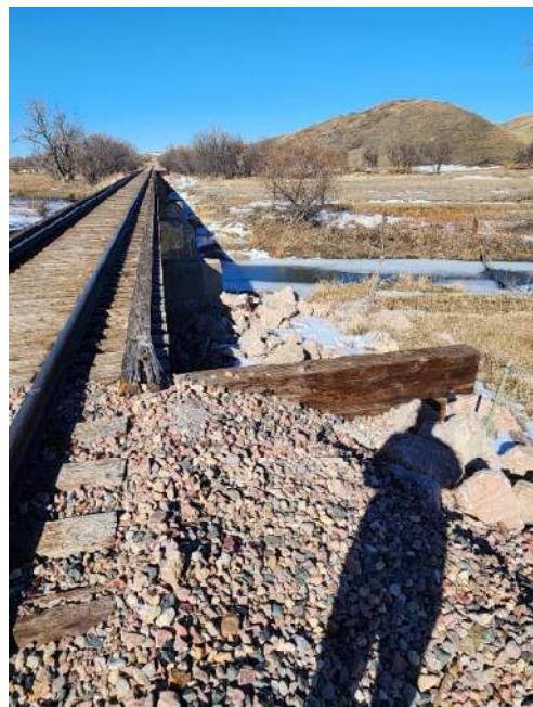
CDI_Channel Looking Northwest Downstream of Bridge at MP 617.30
