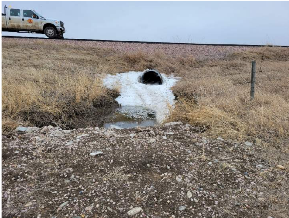
CDI_Downstream End of Existing 48" CMP
