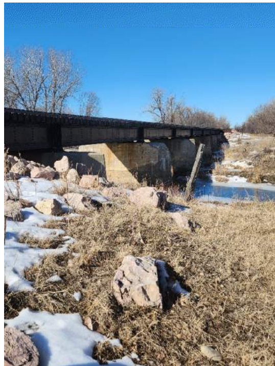
CDI_Profile Structure 617.30 Looking Southwest
