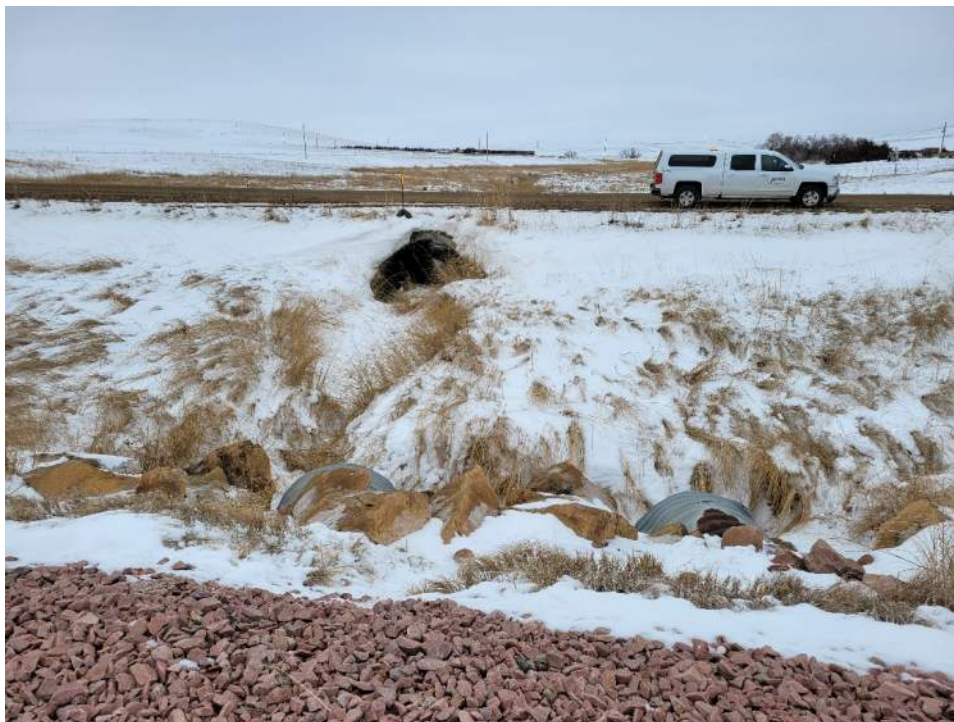
CDI_Upstream Looking North at Bad River Road & Ex. 96" RCP Arch
