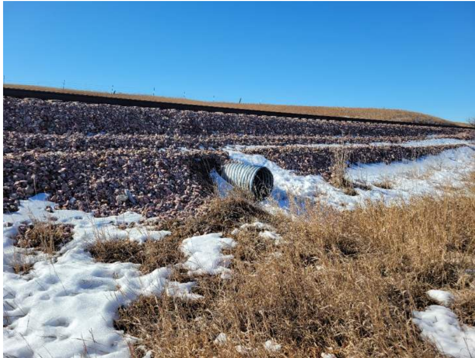
CDI_Downstream End of Existing 24" CMP
