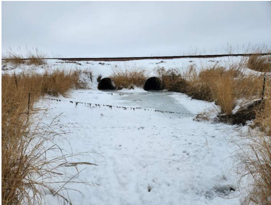
CDI_Downstream End of Existing 2 - 60" CMP
