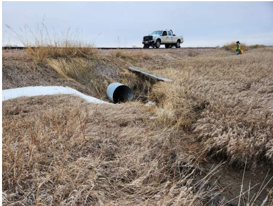
CDI_Upstream End of Existing 48" CMP
