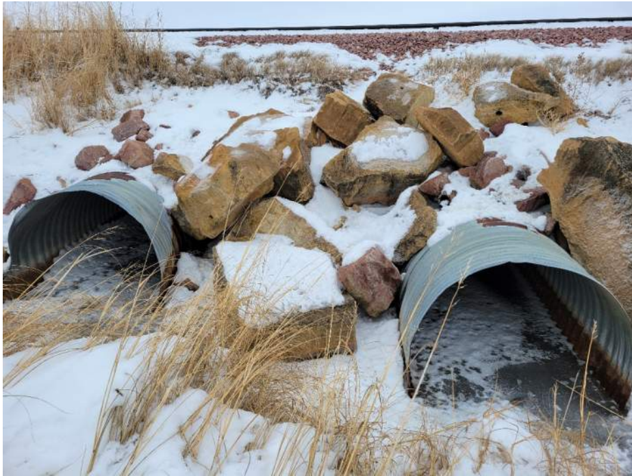
CDI_Upstream End of Existing 2 - 60" CMP
