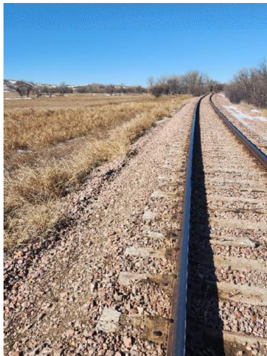
CDI_Looking West Upstream of Grant Application Structure Location (MP 617.15)
