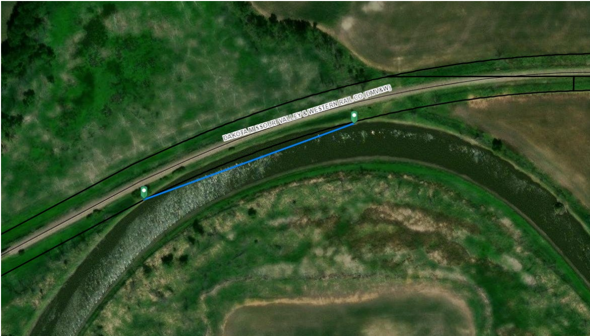
Satellite image showing approximately 600 feet of riverbank eroding close to the railroad grade.
