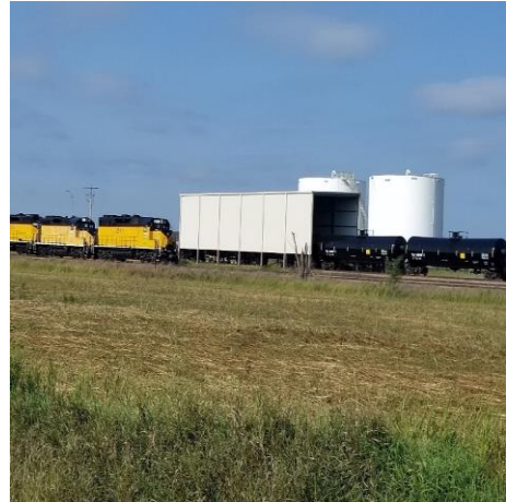
Figure 4: D & I at Siouxland Energy Cooperative located at Hudson, South
