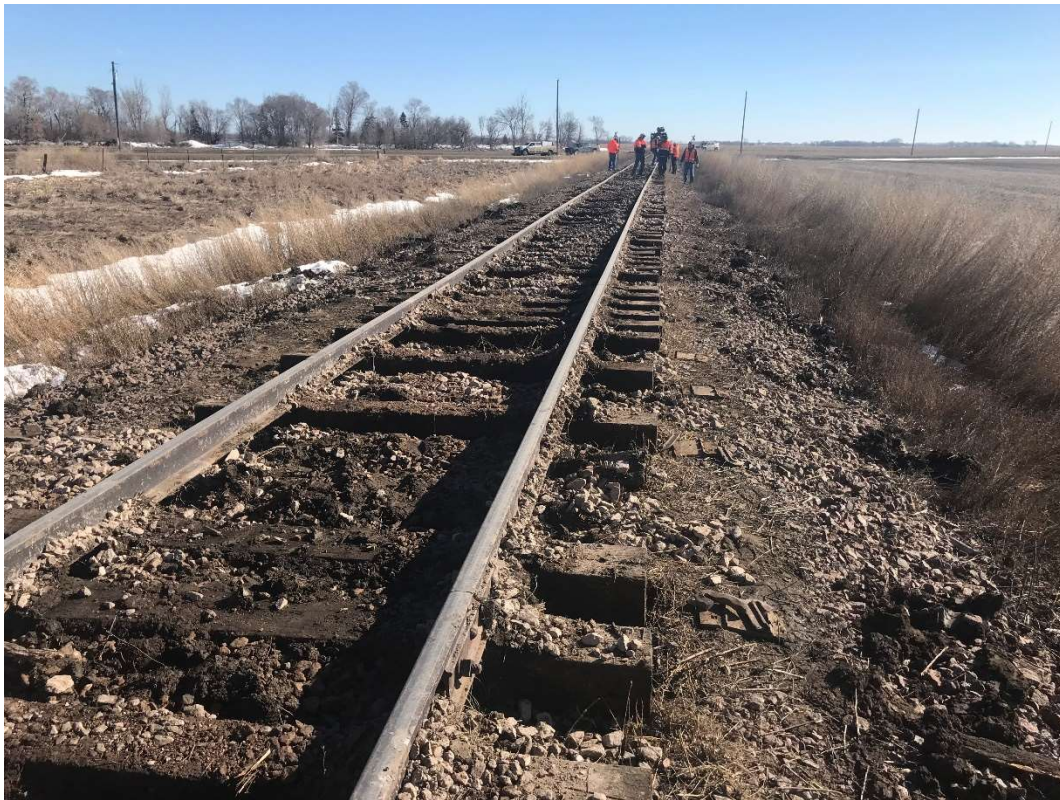
Example of Poor Subgrade and Tie Conditions
