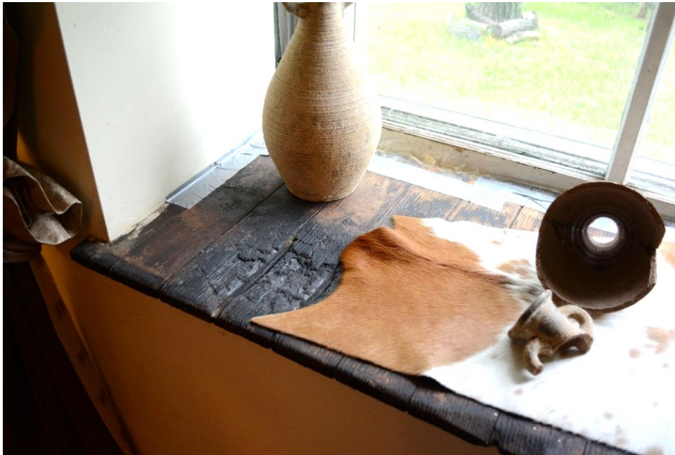
ClarkCounty_Klampe-MannHouse_0016.JPG Living room windowsill, detail of burn damage. Date: June 27, 2024
