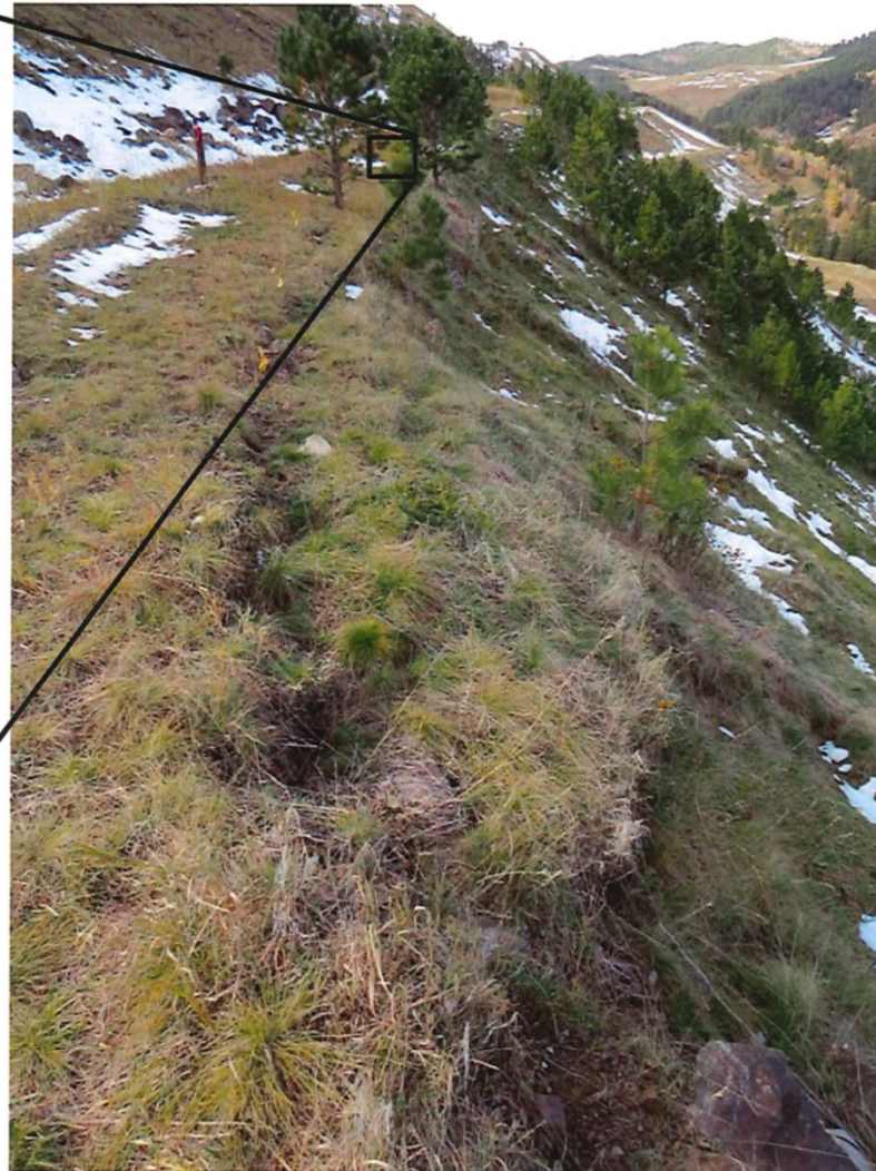
TENSION CRACK AT THE CREST OF THE 5100 BENCH IN GAYVILLE GULCH LOOKING WEST (PHOTOGRAPH TAKEN ON OCTOBER 17, 2019)
