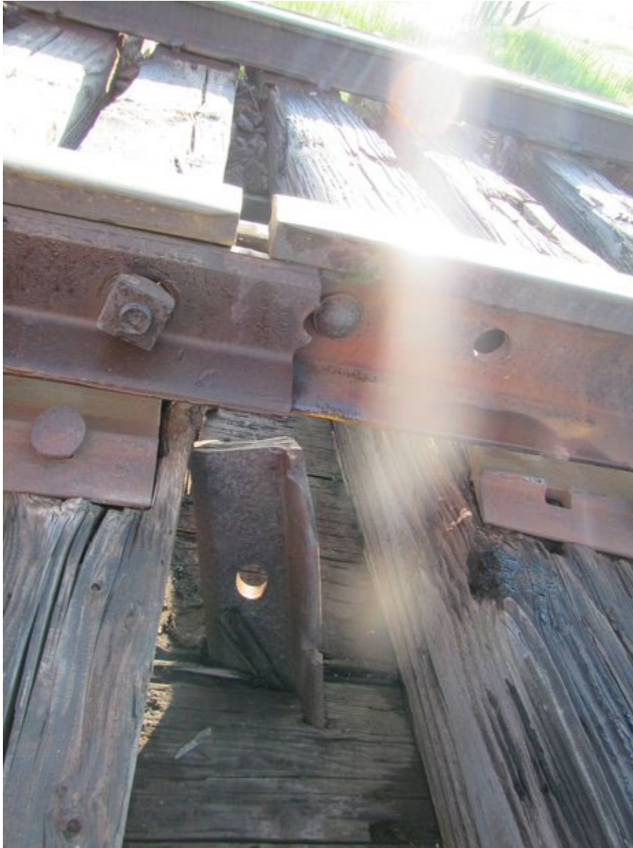
Broken joint bar
