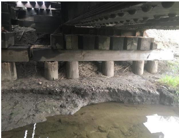
Figure 4: Bridge T512.5 Bent #3 mainline, reflecting hollow pile, remaining poor caps with one missing, splitting caps
