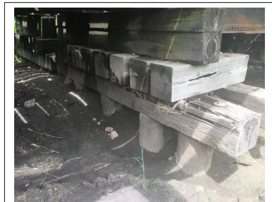
Figure 3: Bridge T512.5 Bent #2 showing checking on the cross cap, rotting pile
