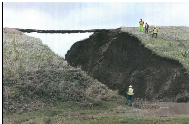
RCP&E lost of culvert at Van Metre SD
