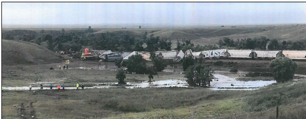
Wide angle view shortly after loss of culvert at New Underwood SD and subsequent derailment, note locomotives on the left of the derailment with lead locomotive out of sight on its side
