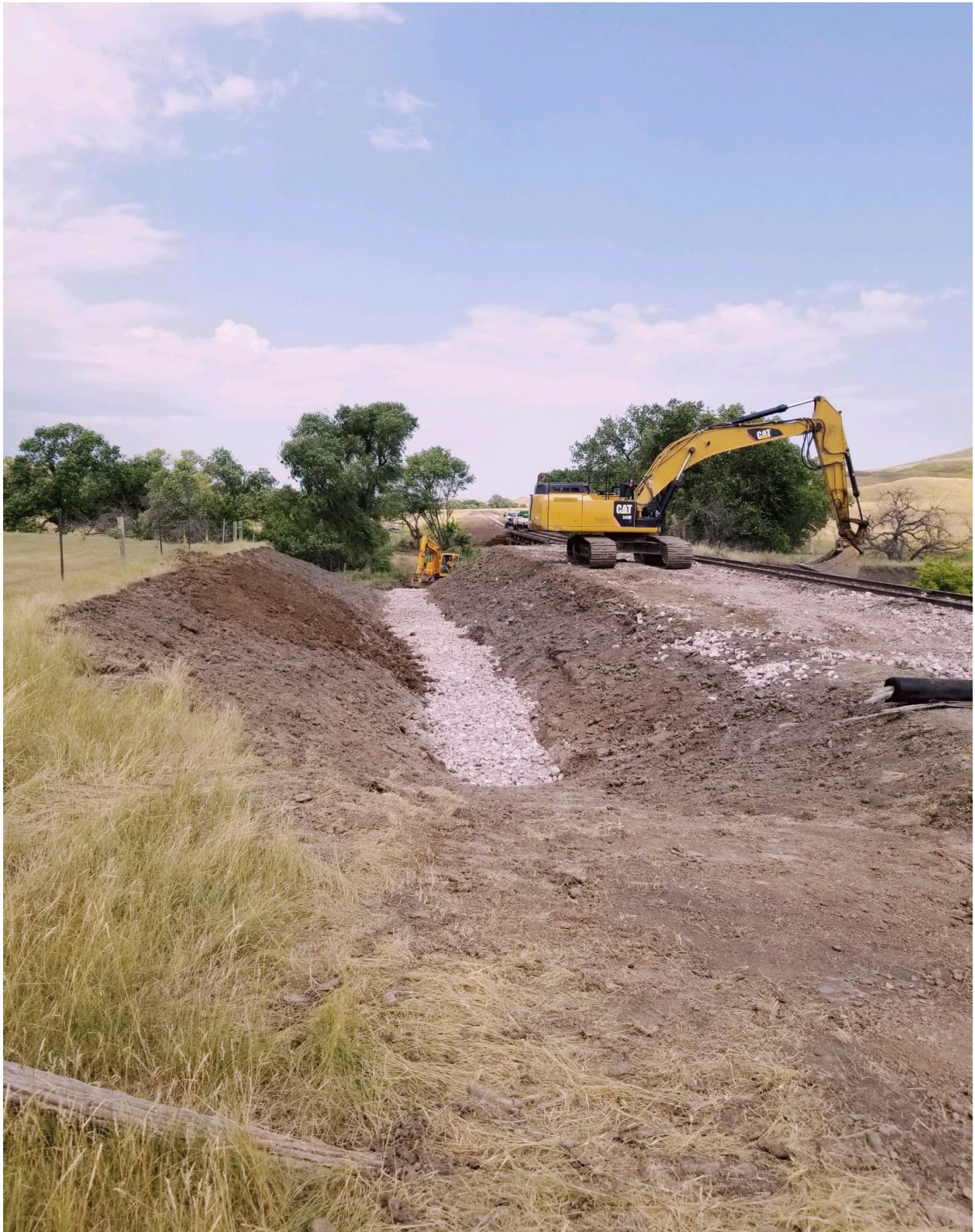
Mp 448.5 French drain installation 8-25-22
