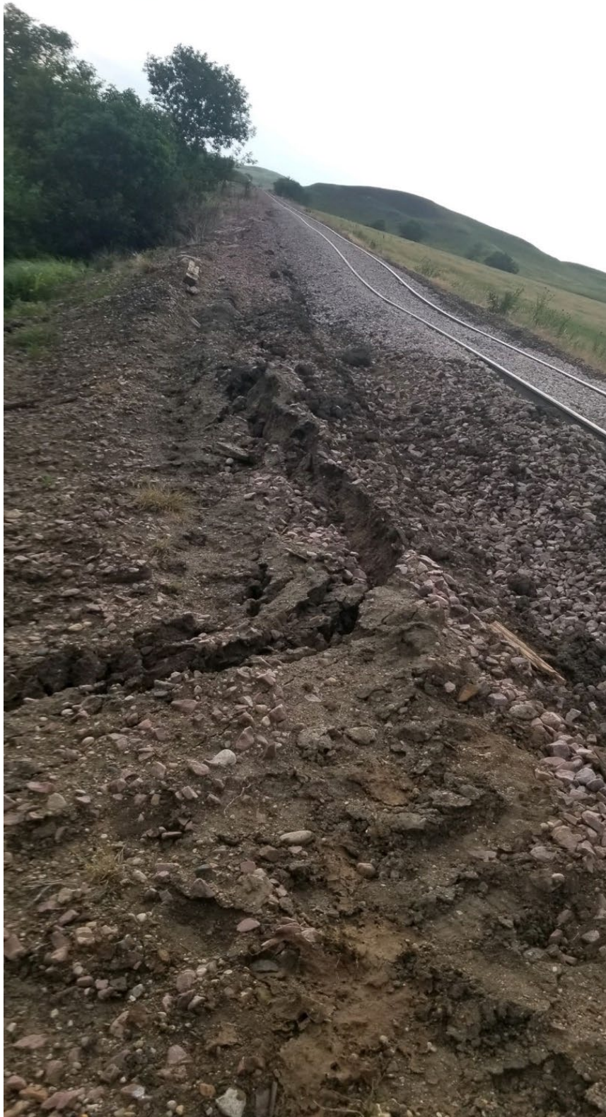
Embankment failure west river
