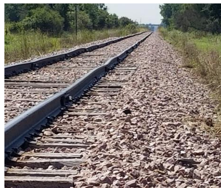
Figure 5: Existing D & I Track Condition with Bent Rail Ends and Rail Warp
