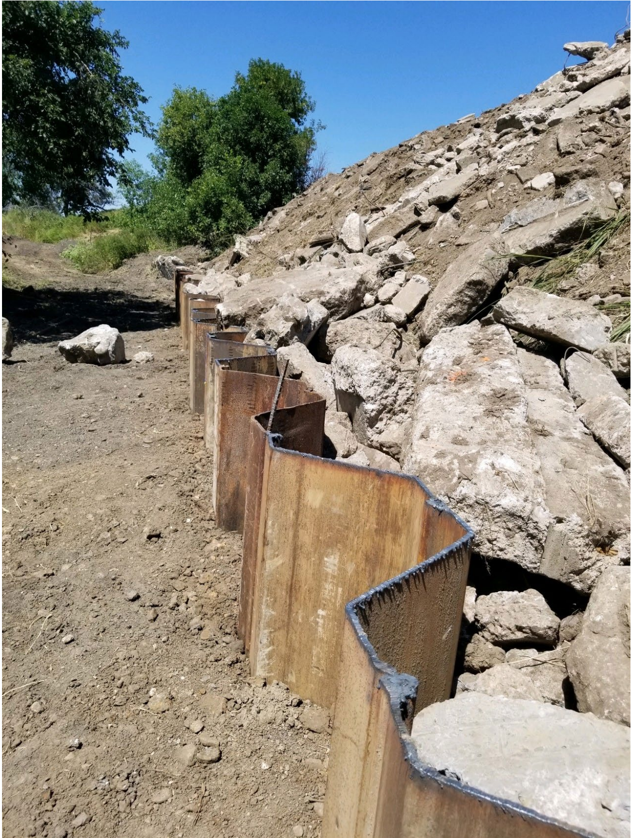
Sheet pile and embankment repair 8-10-22
