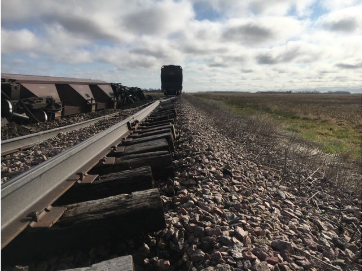
2020 Derailment – soft subgrade/poor tie condition
