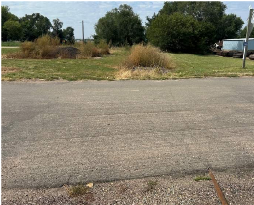
Figure 7 – Railroad Crossing in Tabor that has been paved over with asphalt.
