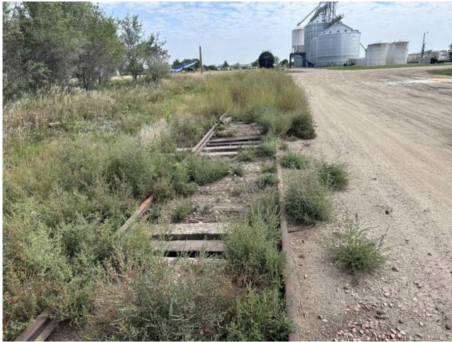
Figure 6 – Track condition in east Tabor (MP 10.0 to MP 10.4) with empty cribs and brush overgrowth.
