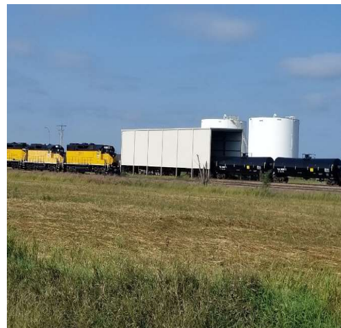
Figure 4: D & I at Siouxland Energy Cooperative located at Hudson, South
