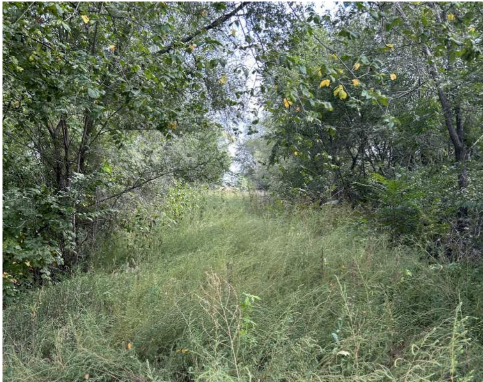
Figures 8 & 9 – Brush overgrowth on track in west Tabor (MP 10.4 to MP 10.9).
