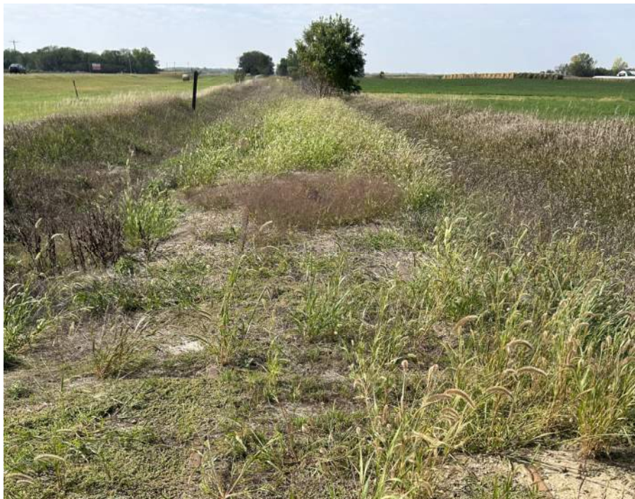
Figures 10 & 11 – General track condition from west Tabor (MP 10.9) to MP 14.5.
