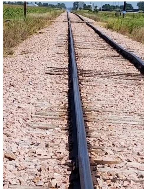
Figure 4: Existing Condition Showing Surface of Track on the D & I Railroad line
