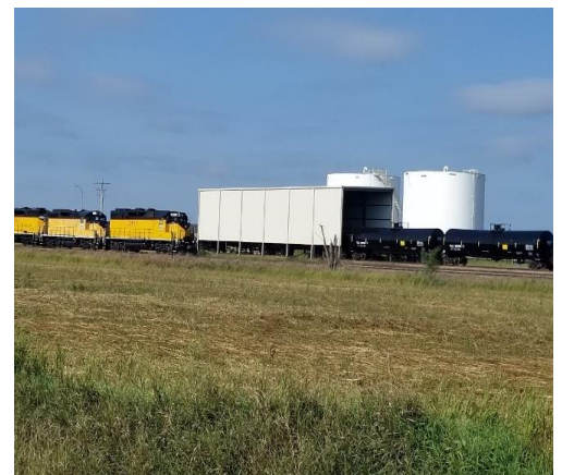
Figure 3: D & I at Siouxland Energy Cooperative located at Hudson, South
