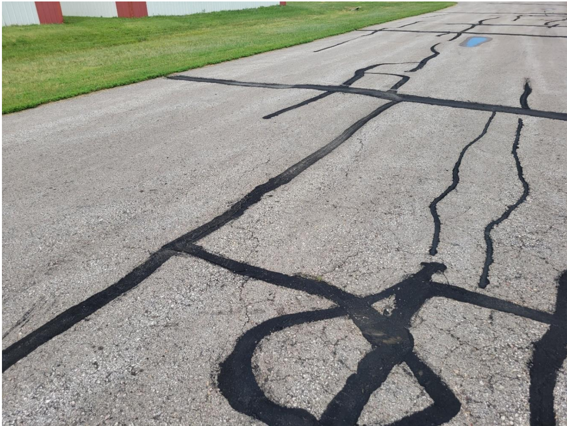
Exhibit 1 - Taxilane after pavement maintenance. Pavement alligator cracked.
