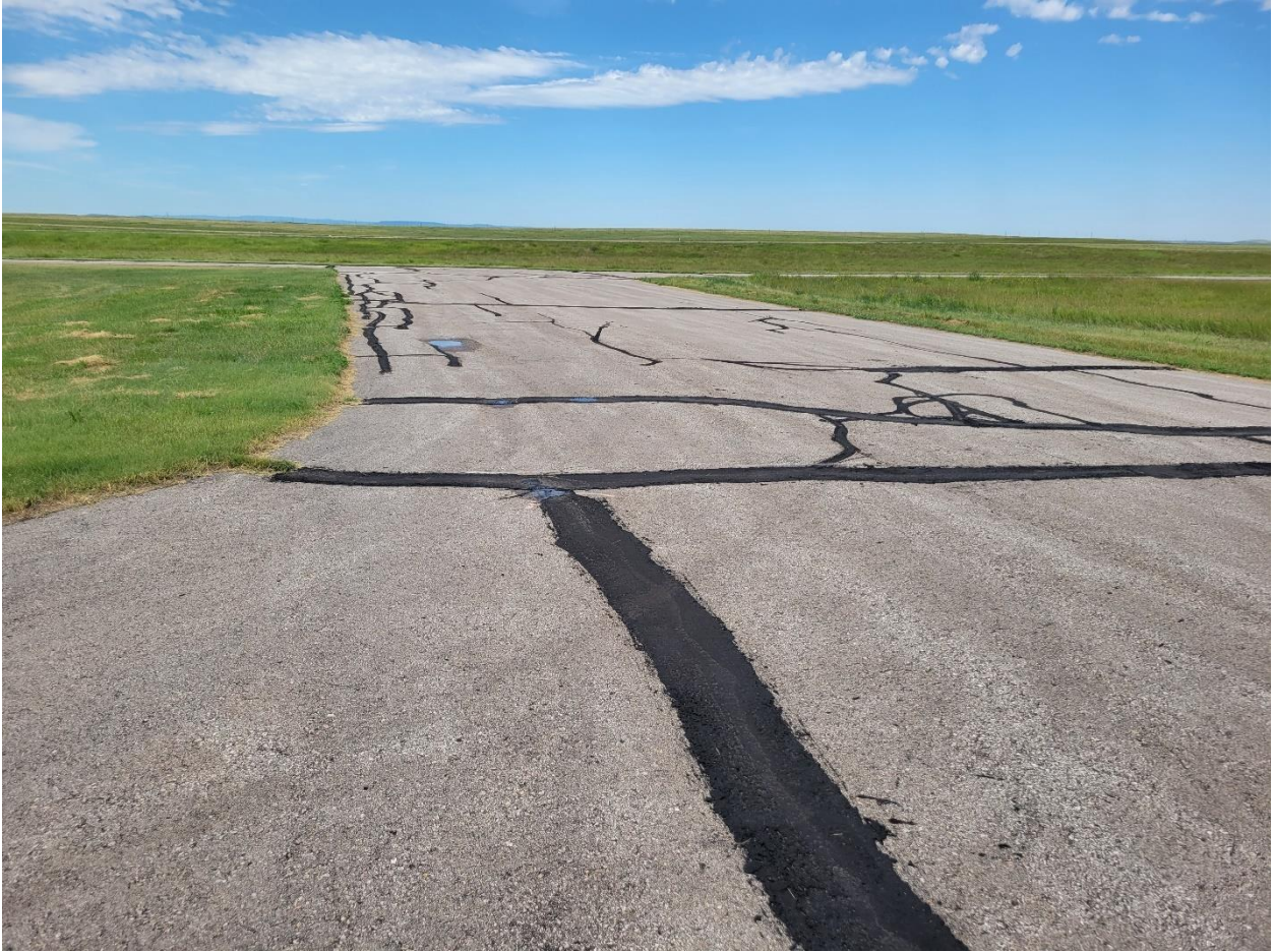
Exhibit 2 - Taxilane after pavement maintenance.
