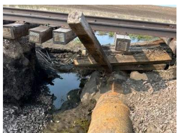
Figures 6 - 11 – Track washouts resulting from flooding during spring of 2023.
