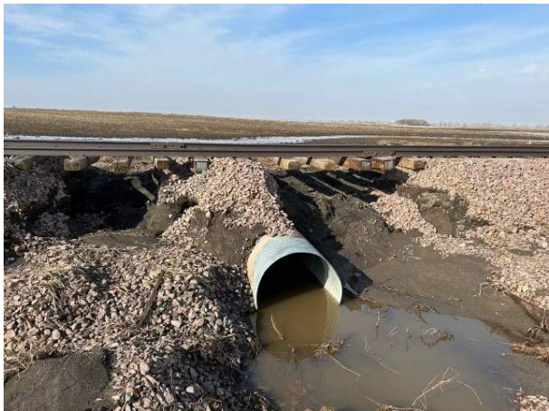
Figures 6 - 11 – Track washouts resulting from flooding during spring of 2023.
