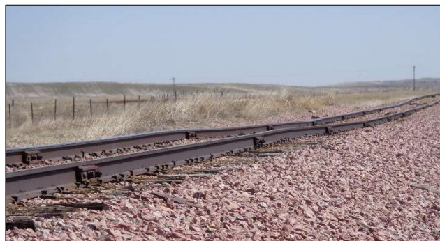
Typical section of 100 year old, 100 lb. stick rail on the Fort Pierre – Rapid City line, showing end of rail deflection and rail damage, exacerbated by the Pierre Shale subgrade.
