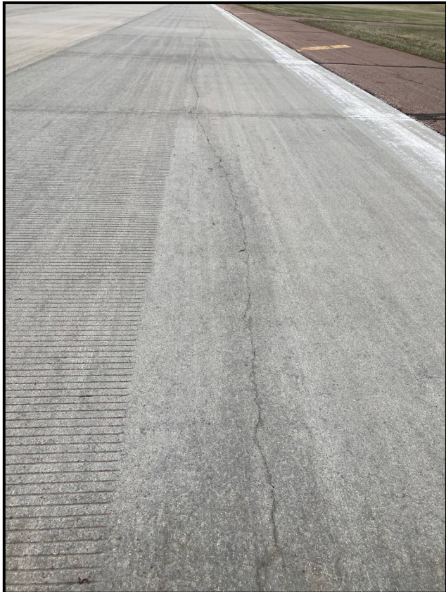
Left: Linear cracking through multiple panels. Right: Particularly bad spall with FOD. Linear crack through panels with joint seal no longer working effectively.
