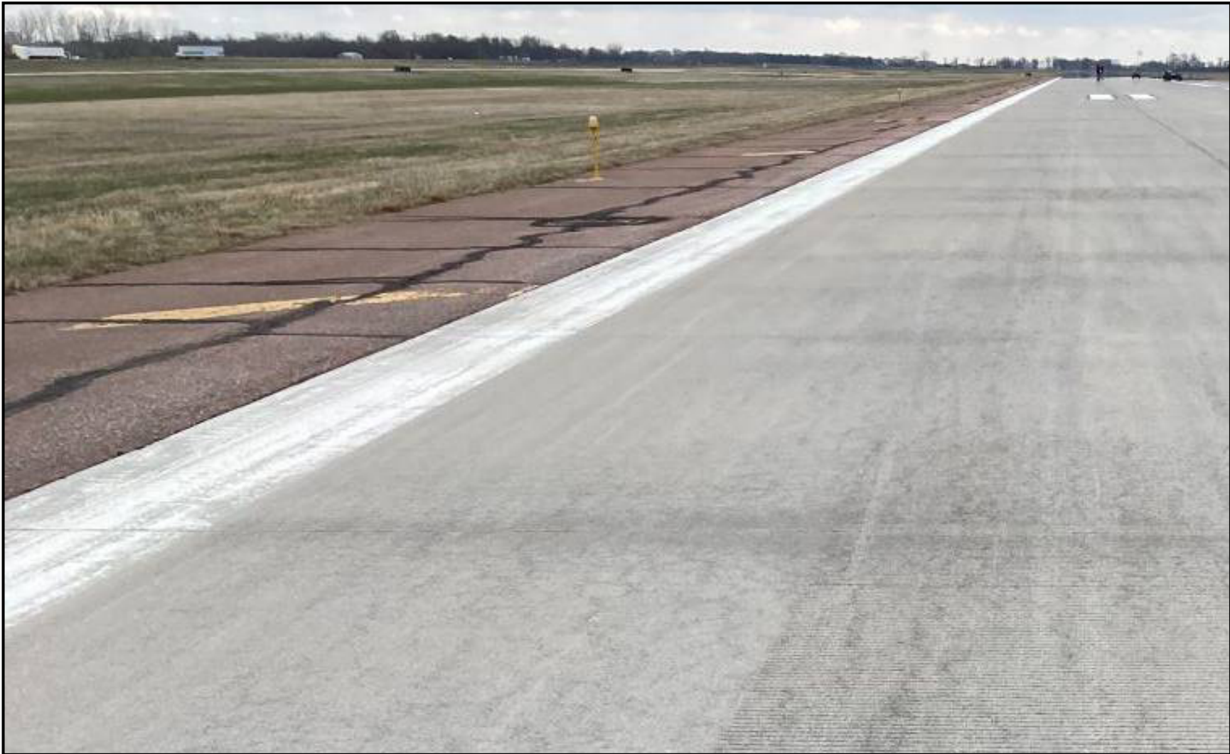
View of Shoulders along the Runway
