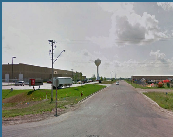
Lennox Industrial Park Improvements
