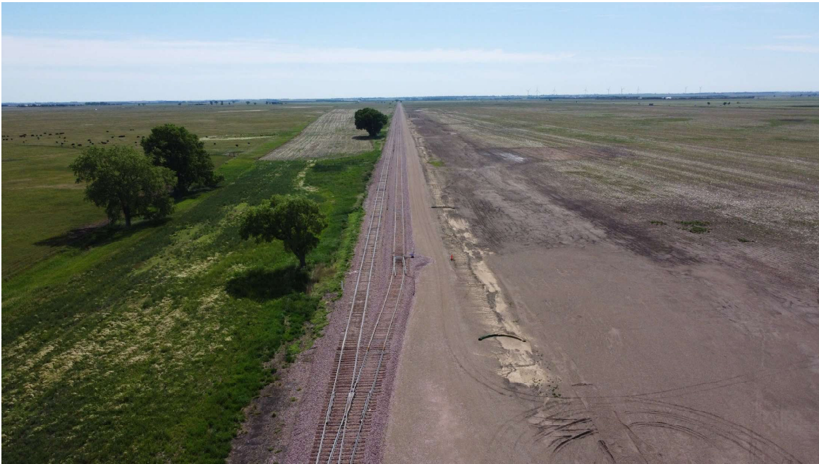
The aerial picture above is the STC 2020 RWRR Meet & Pass Siding
