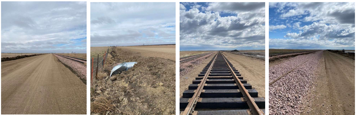
The pictures above are the grade work and track installation STC 2020 RWRR Meet & Pass Siding
