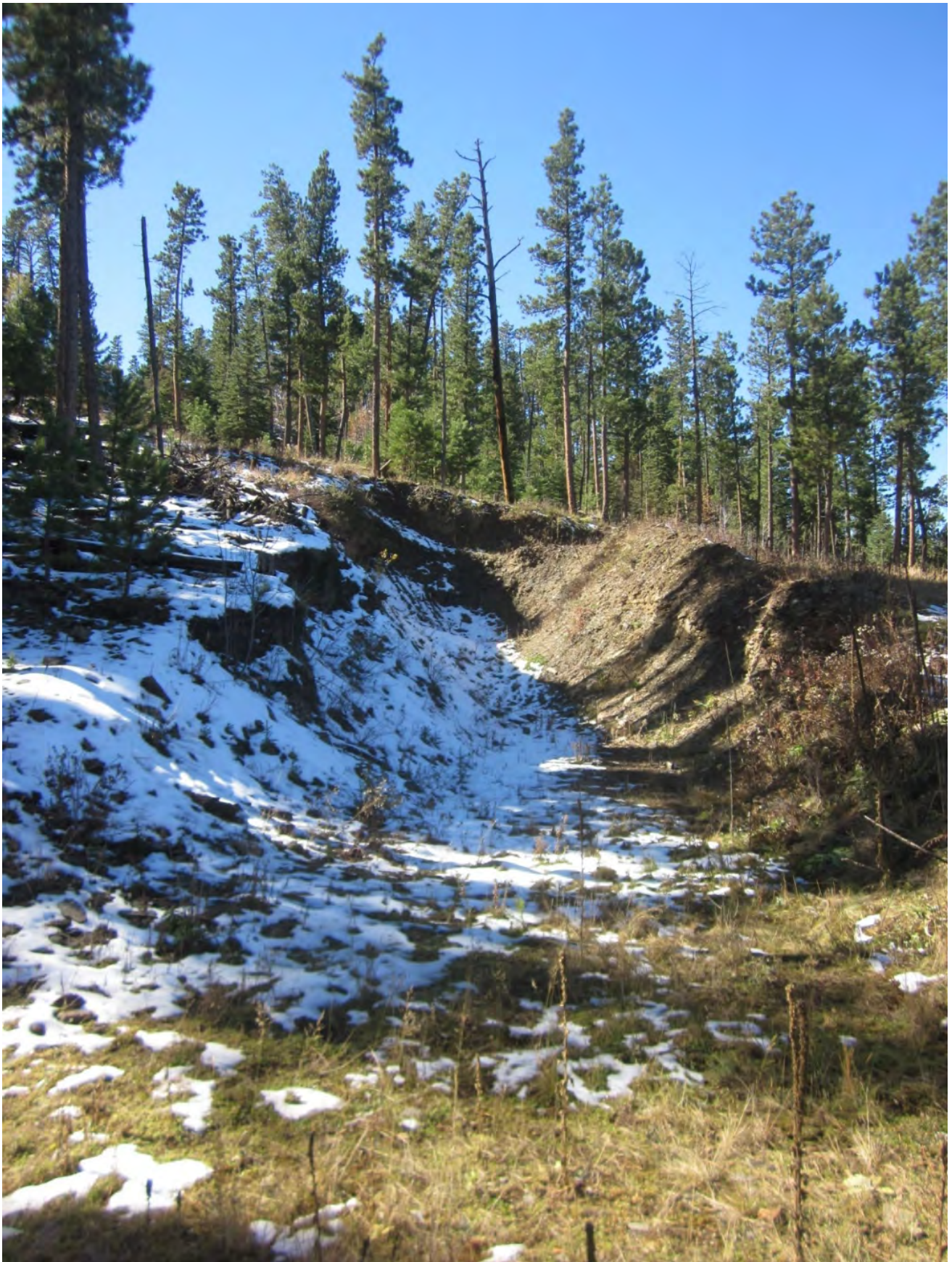
Photo 1. Exploration trench prior to reclamation,
