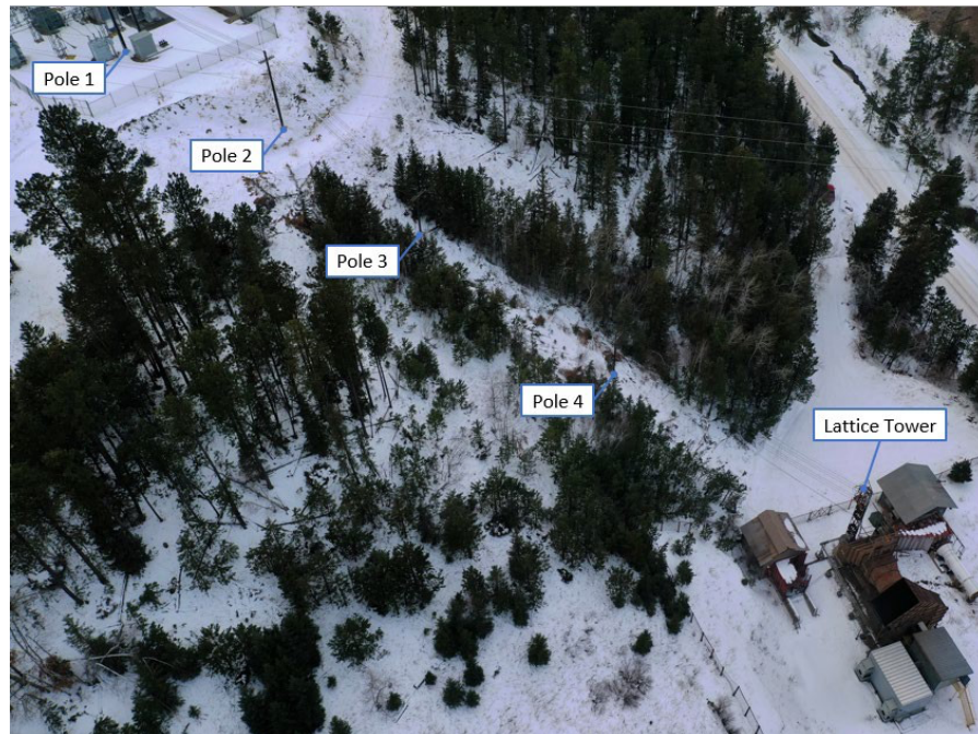
Figure 5.2 – Existing Overhead Line Feeding the OHFC
