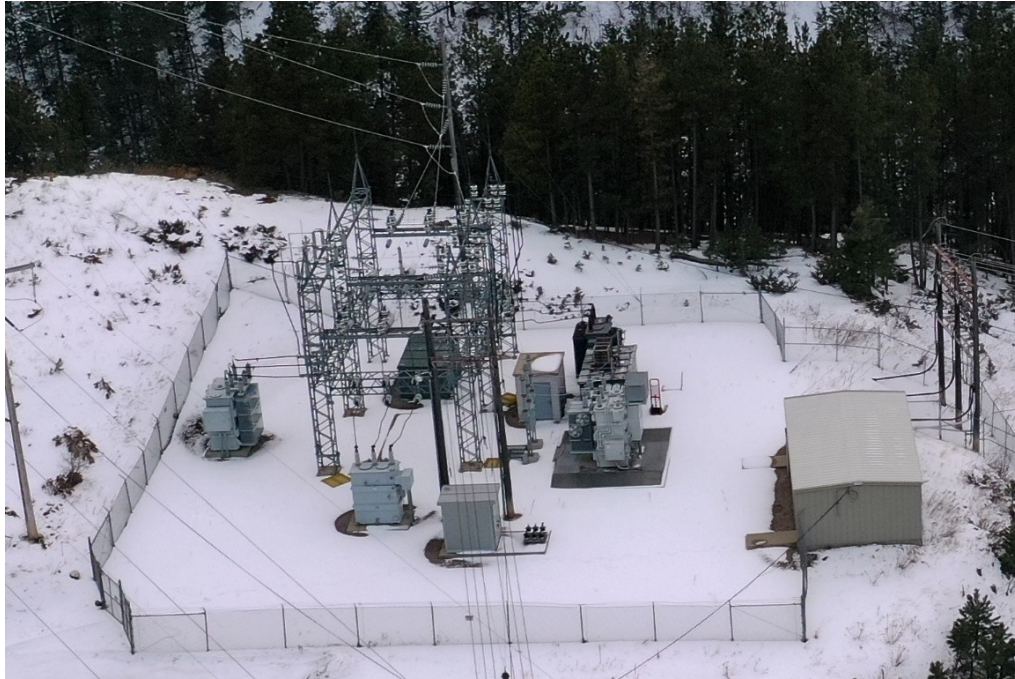
Figure 5.1 - Oro Hondo Substation
