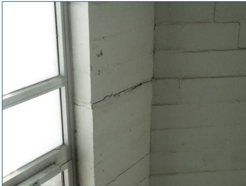
Figure 1-west hall structural fatigue
