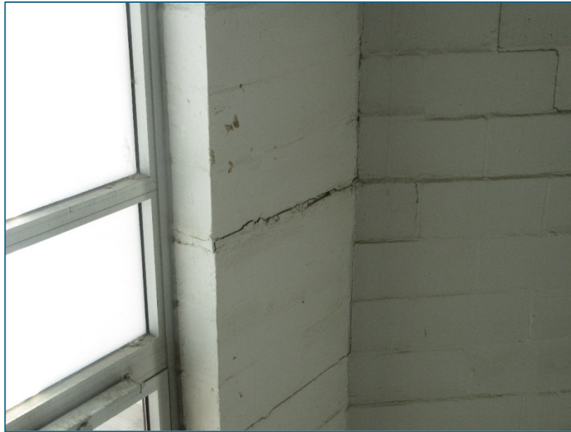
Figure 1-west hall structural fatigue
