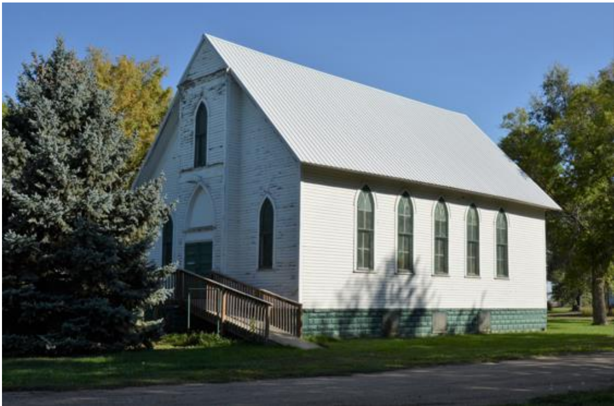
SD_Jerauld County_Zion Emmanuel Lutheran_0001 Exterior of west façade and south elevation, camera facing northeast.
