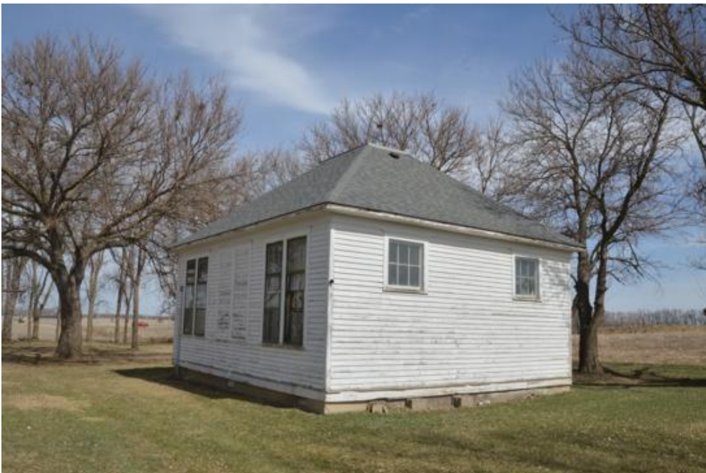
SD_Lincoln County_Sunnyside School No 56_0003 View of west and south elevation, camera facing northeast.
