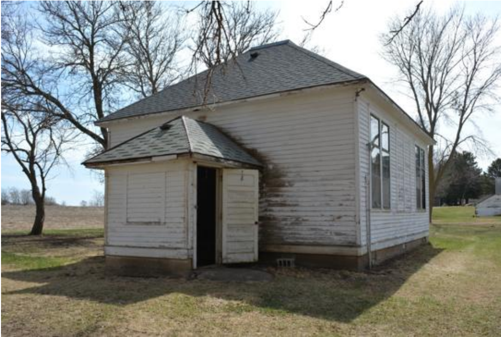
SD_Lincoln County_Sunnyside School No 56_0002 View of north and west elevation, camera facing southeast.
