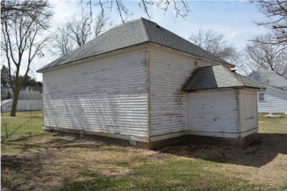
SD_Lincoln County_Sunnyside School No 56_0004 View of east and north elevation, camera facing southwest.
