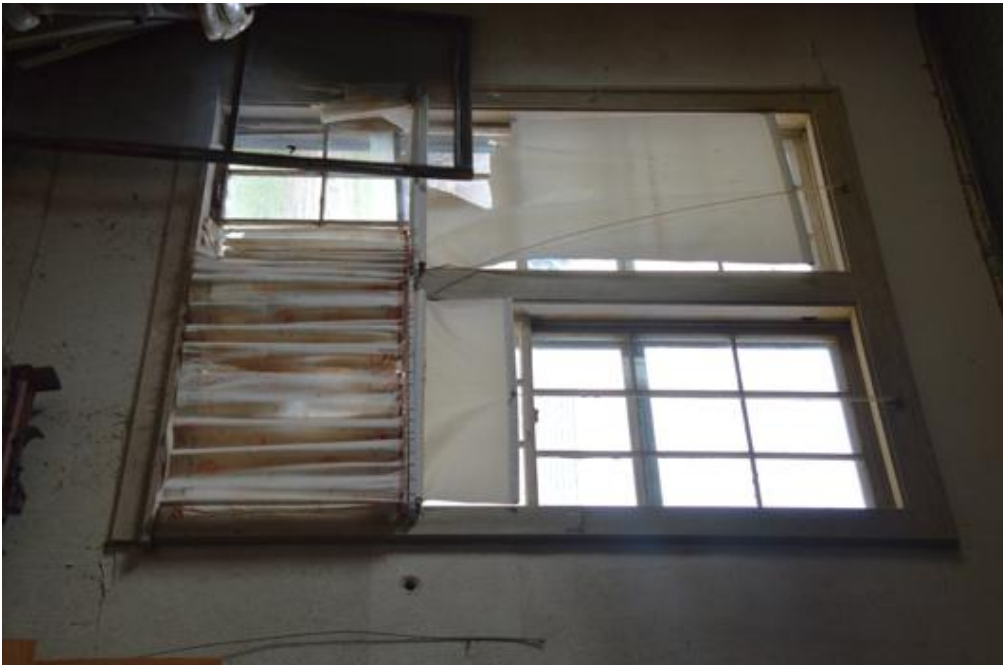
SD_Lincoln County_Sunnyside School No 56_0011 View of classroom windows interior, camera facing southwest.
