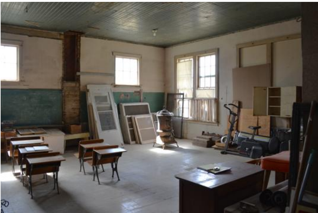
SD_Lincoln County_Sunnyside School No 56_0007 View of classroom interior, camera facing southwest.
