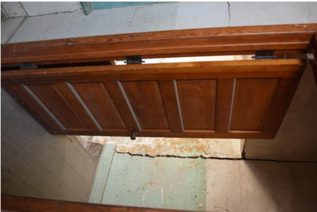
SD_Lincoln County_Sunnyside School No 56_0013 View of classroom entrance to vestibule, camera facing northeast.
