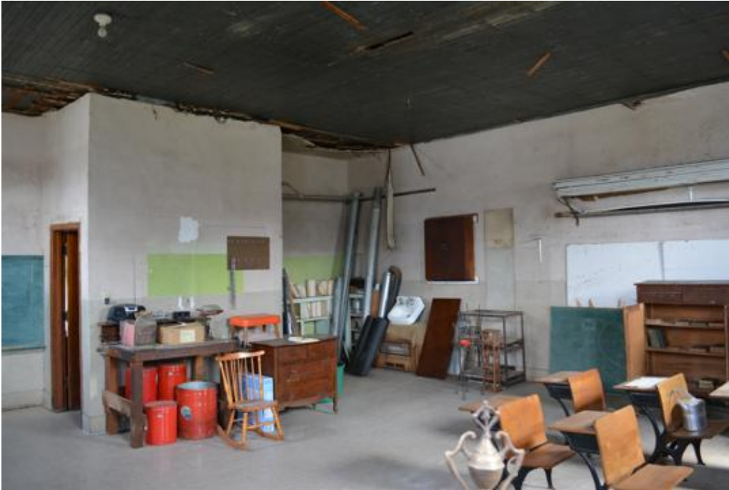
SD_Lincoln County_Sunnyside School No 56_0008 View of classroom interior, camera facing northeast.
