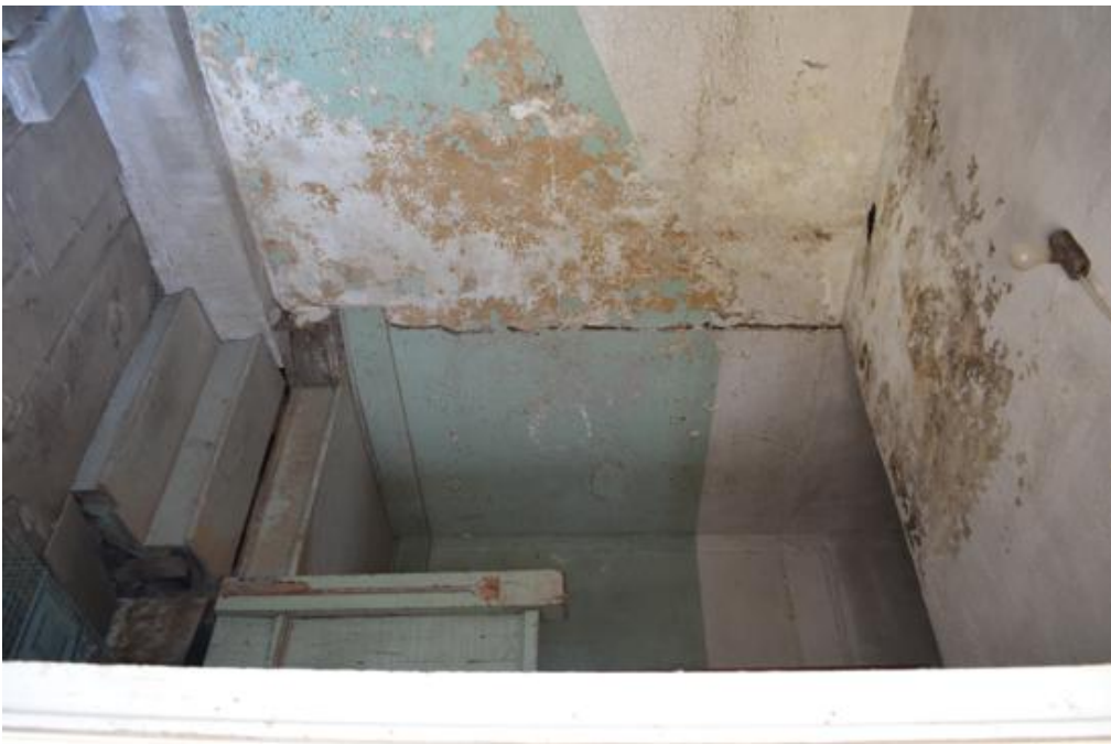
SD_Lincoln County_Sunnyside School No 56_0005 View of entrance vestibule, camera facing southeast.
