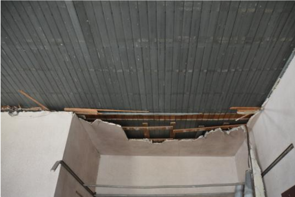
SD_Lincoln County_Sunnyside School No 56_0010 View of classroom ceiling, camera facing north.
