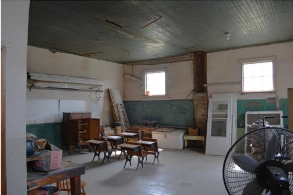
SD_Lincoln County_Sunnyside School No 56_0006 View of classroom interior, camera facing southeast.
