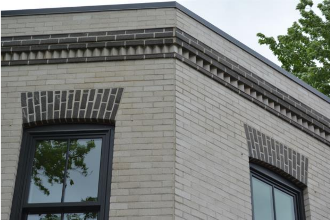
SD_MinnehahaCounty_EfftingGrocery_0006 Detail of brick masonry design at window lintels and cornice, camera facing southeast.
