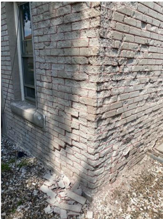
Detail of brick condition and proposed replacement comparison, from the owner in Part 2 application, May 2022.
