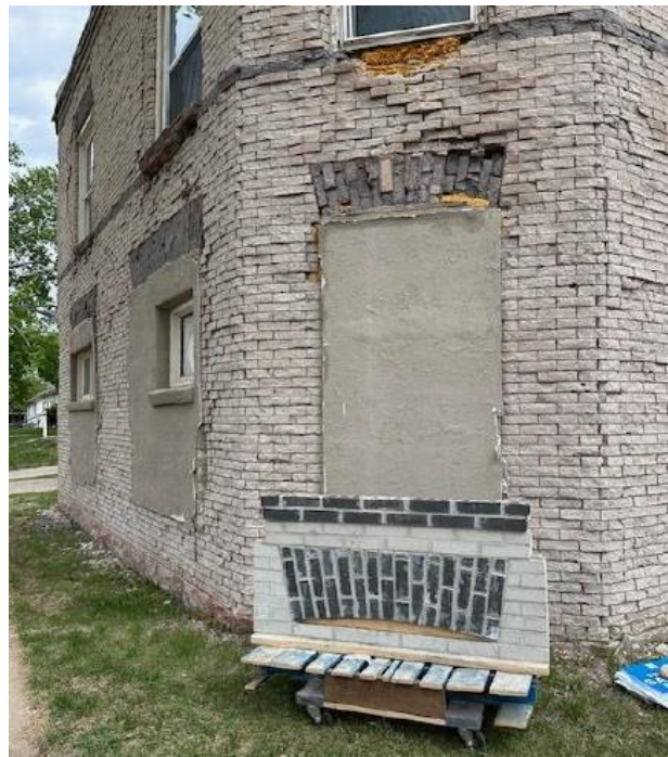
Detail of brick condition and proposed replacement comparison, from the owner in Part 2 application, May 2022.
