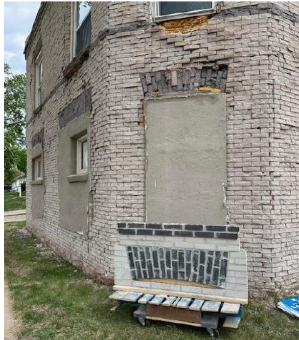
Detail of brick condition and proposed replacement comparison, from the owner in Part 2 application, May 2022.
