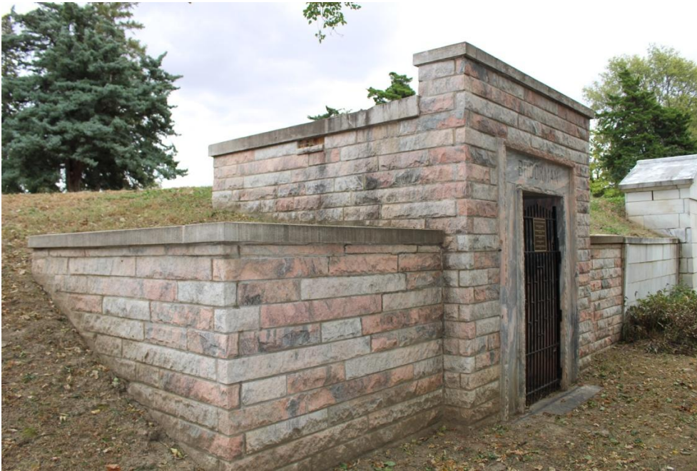
SD_Clay County_Bluff View Cemetery Mausoleum District_0009 Brookman #2 Mausoleum, front and west side, looking northeast.
