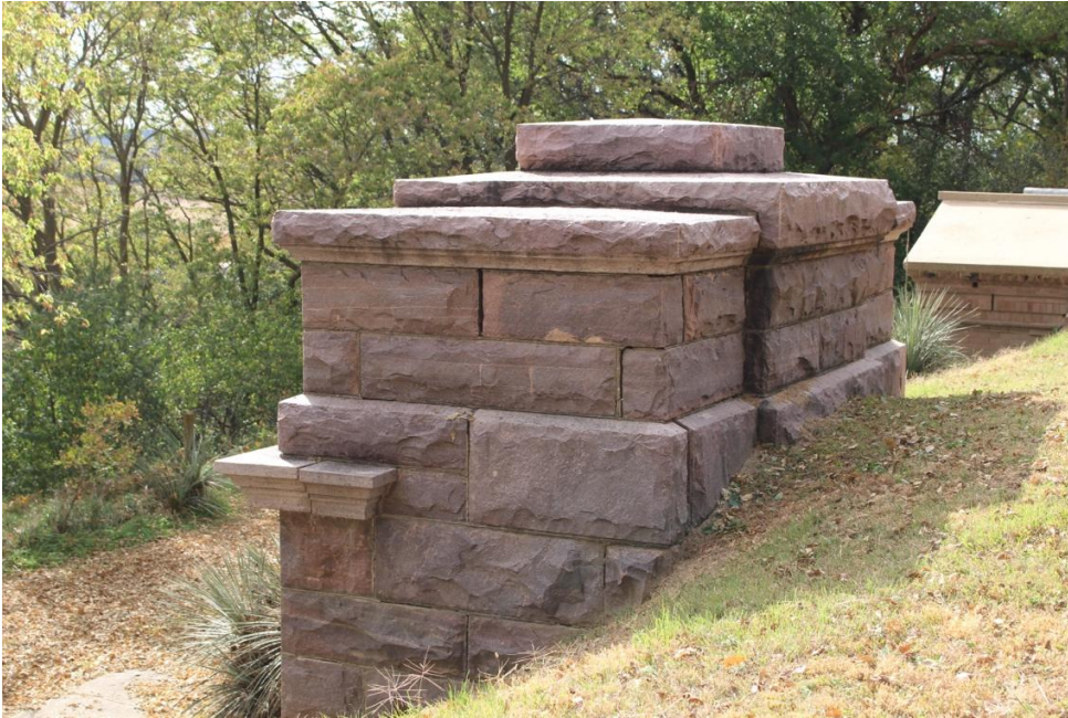
SD_Clay County_Bluff View Cemetery Mausoleum District_0005 Lewis-Thompson Mausoleum, east and rear walls and roof, looking southwest.
