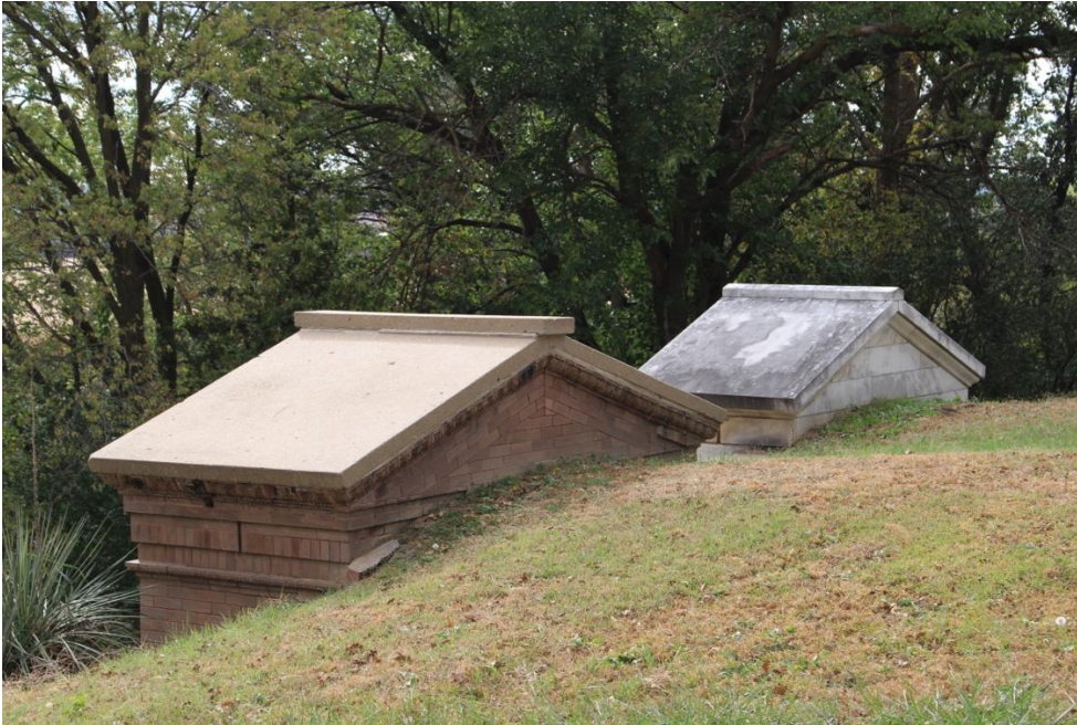
SD_Clay County_Bluff View Cemetery Mausoleum District_0007 Rear and roofs of Brookman #1 Mausoleum (left) and Harrington Mausoleum (right), looking southwest.
