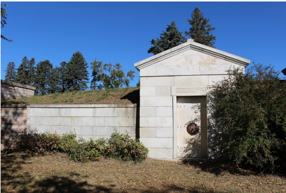
SD_Clay County_Bluff View Cemetery Mausoleum District_0008 Harrington Mausoleum, front, looking north.
