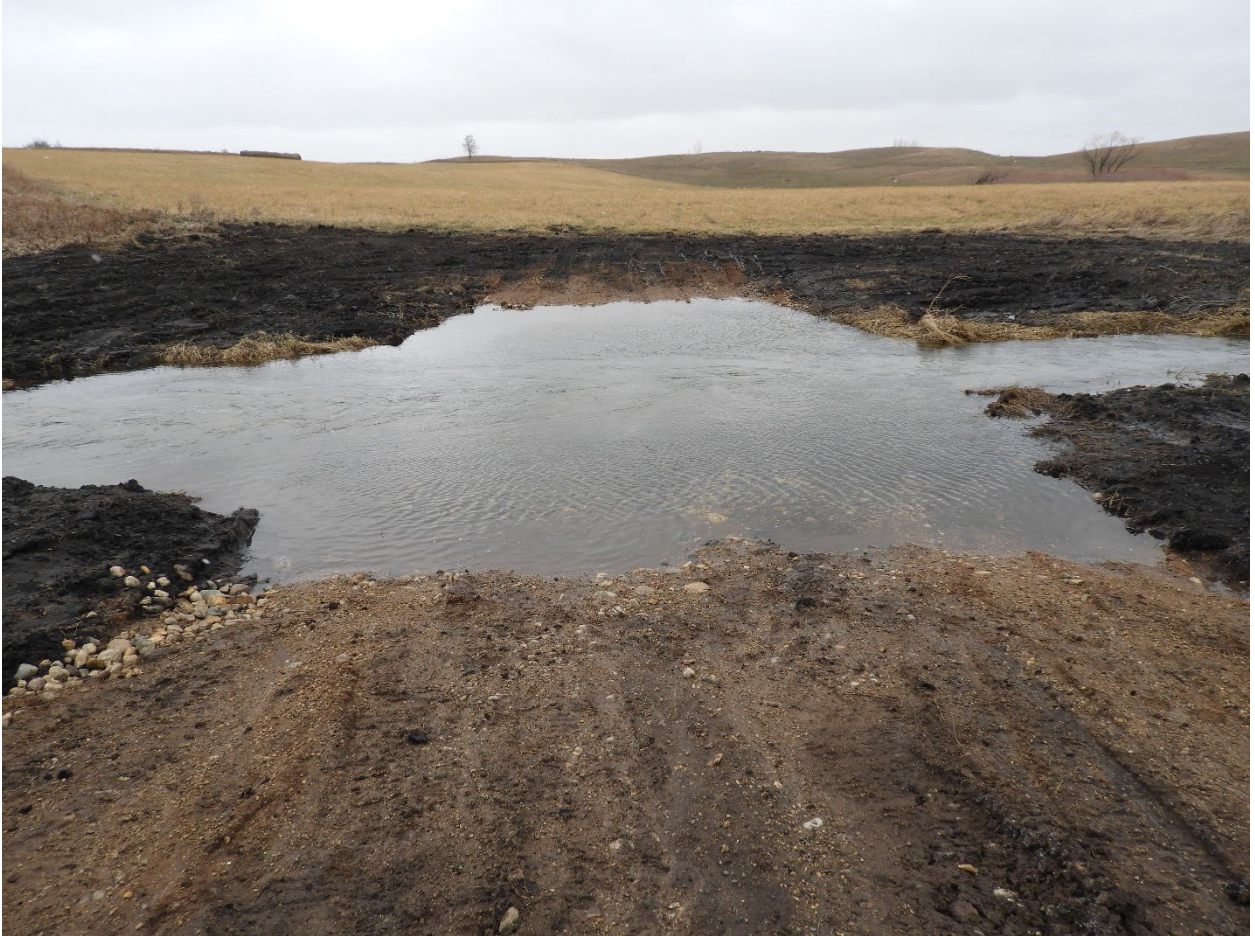
Completed stream crossing Marshall County.
