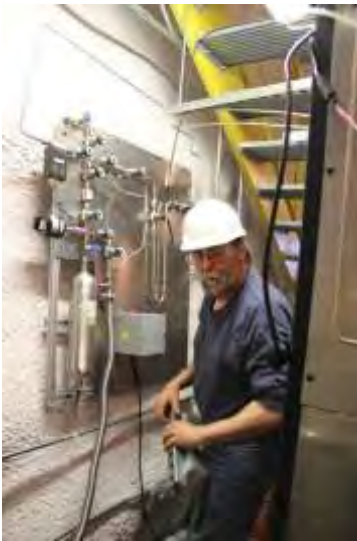
Fig. 1 SDSTA electrician installing outlets for LUX xenon system.
