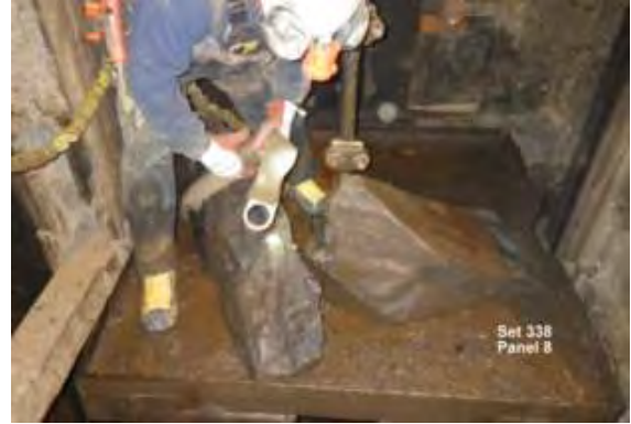
Yates – Infrastructure Technician Removing Rock from Skip
