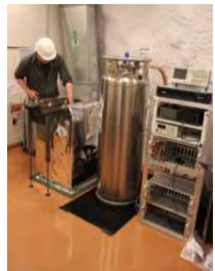
Fig. 5 BLBF system assembled and commissioning underway.
