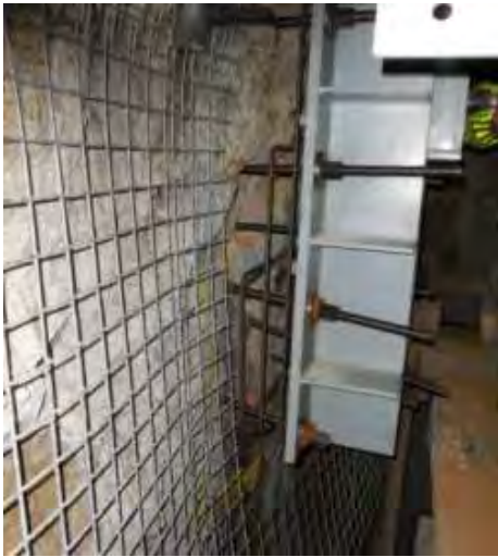
Ross – Rebar Nest Behind Bearing Saddle
