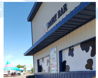
The newly finished Pipestone Discovery Barn at the Sioux Empire Fair includes Midwest Dairy's concession.
