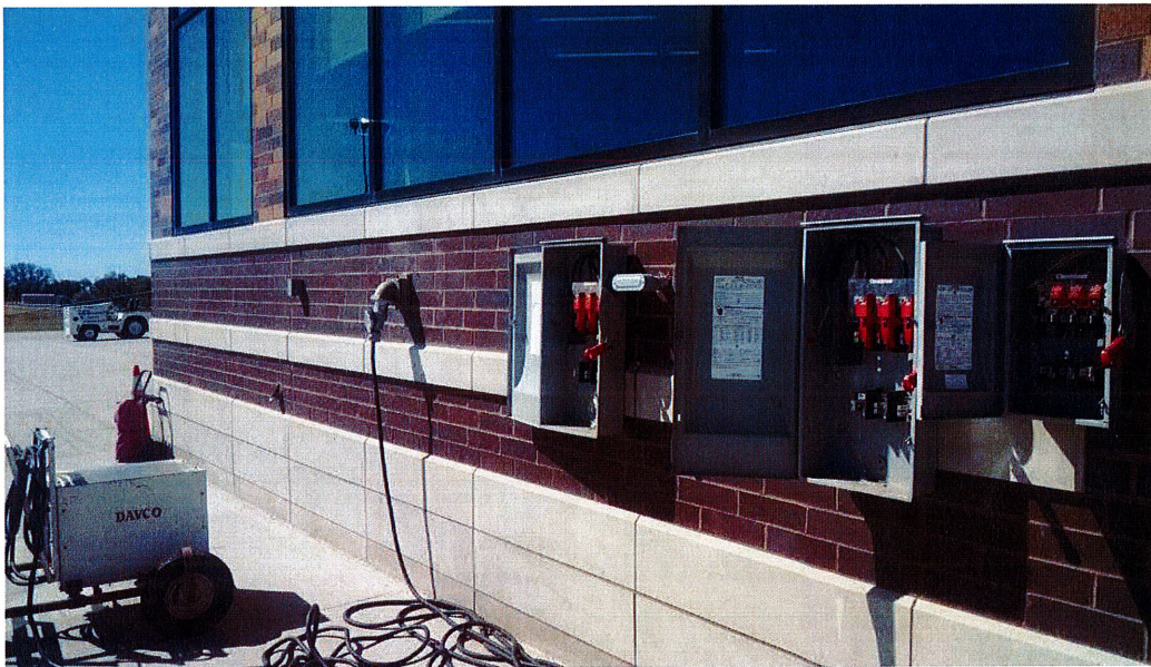
Electrical Provisions for Boarding Bridge
