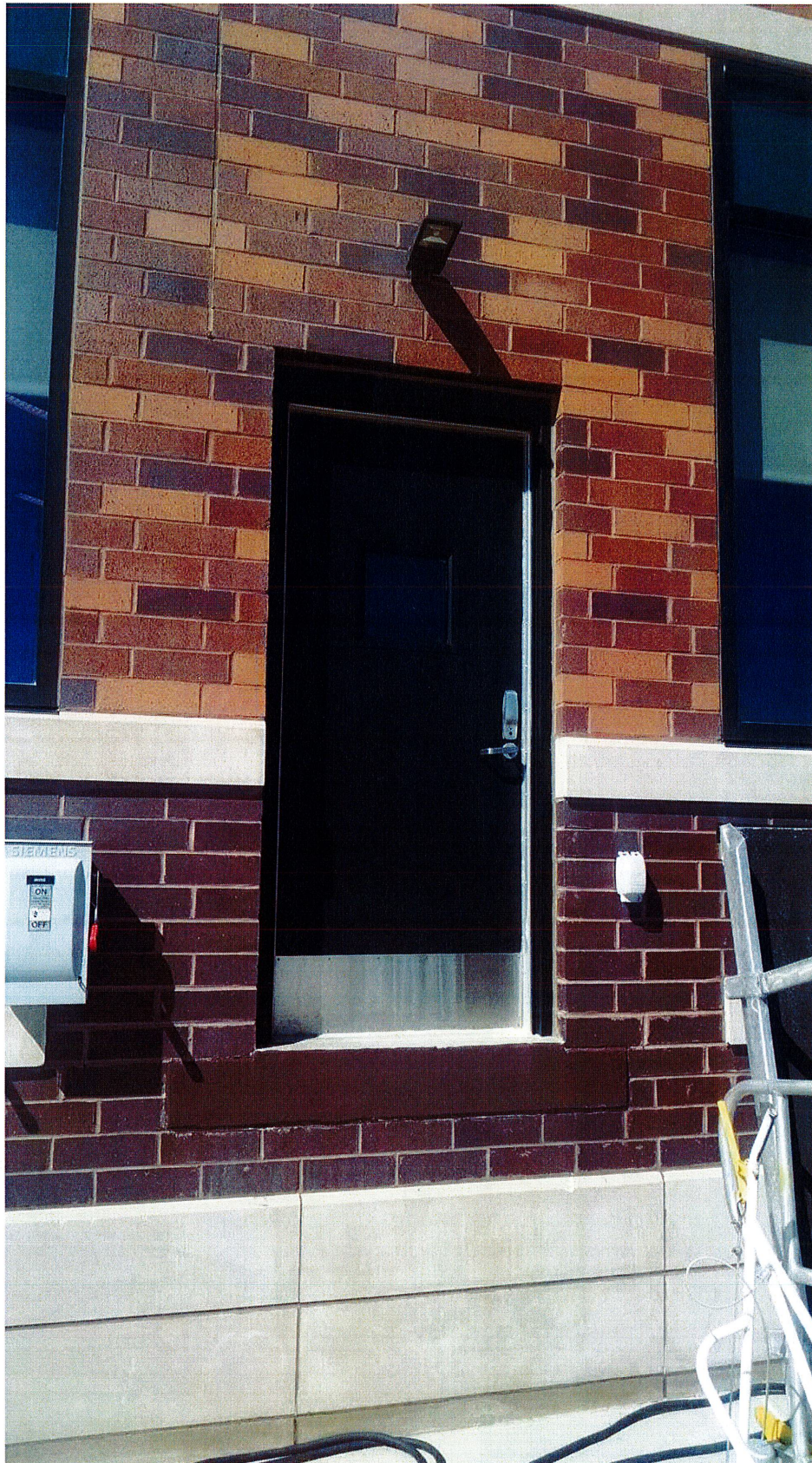
Entrance Door for Boarding Bridge
