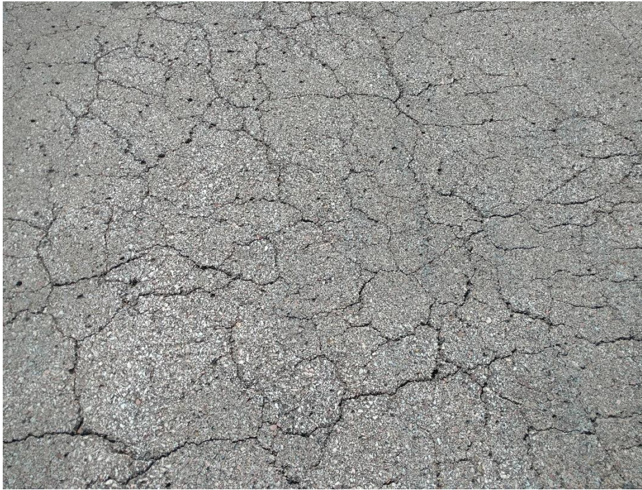
General Aviation Apron. Typical conditions – alligator cracking
