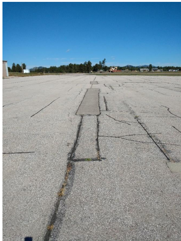
General Aviation Apron. Taken at General Aviation Terminal facing north looking at the Runway 8-26 connecting taxiway.
