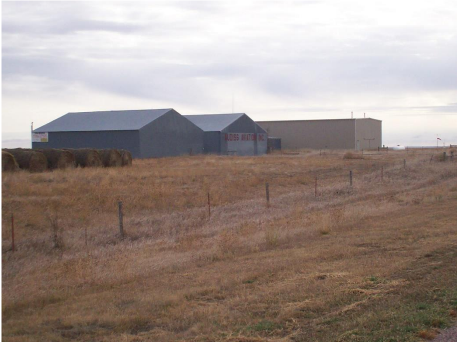
Typical existing fence
