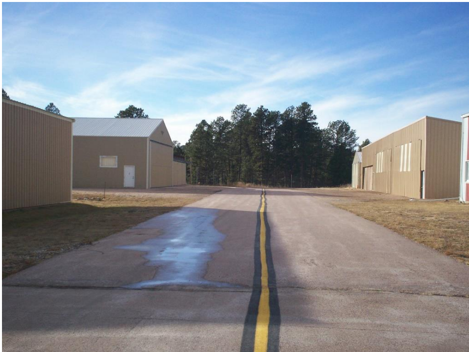
East / West Taxilane – Typical conditions with some ponding water.
