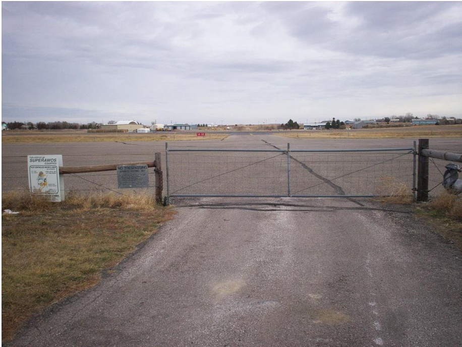
Existing apron access gate
