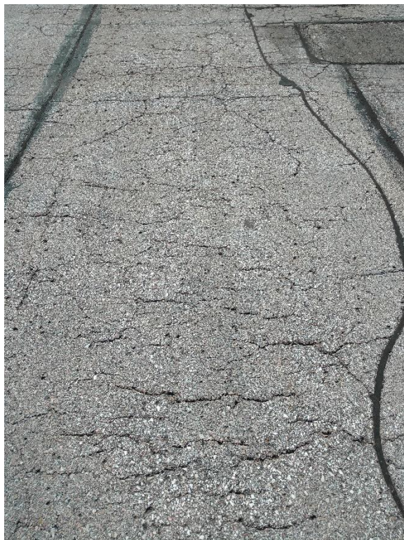
General Aviation Apron – Area of random cracking
