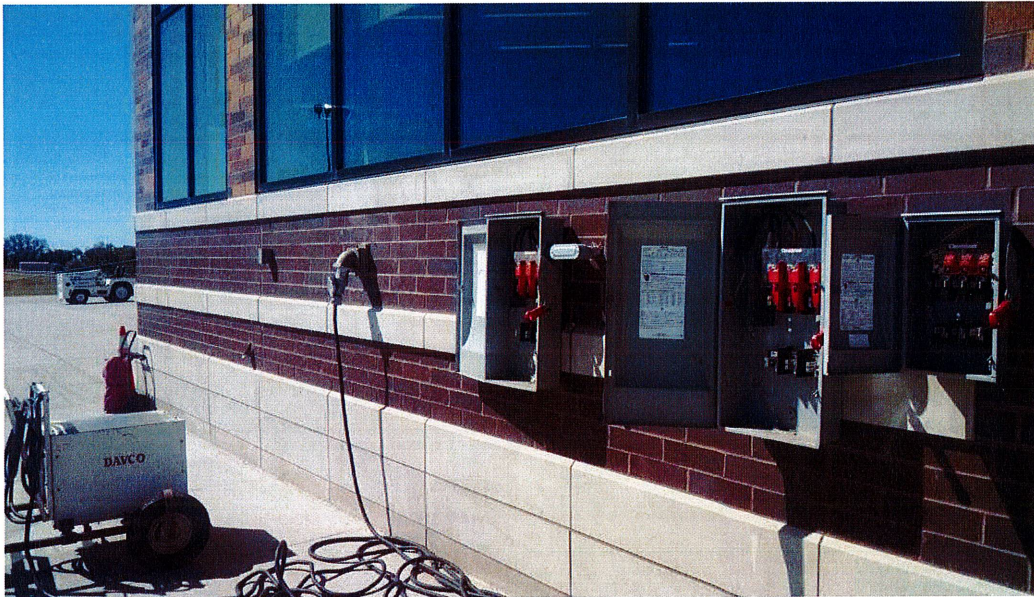
Electrical Provisions for Boarding Bridge
